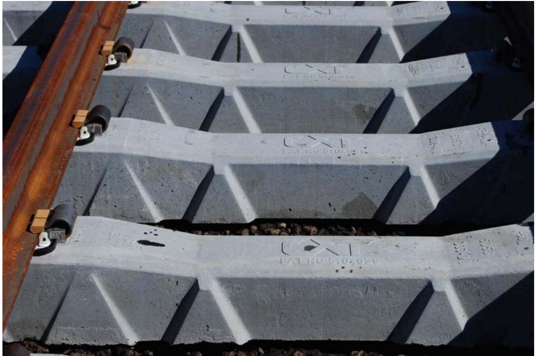
Union Pacific Crenellated Ties Newly Installed at Grand Island
