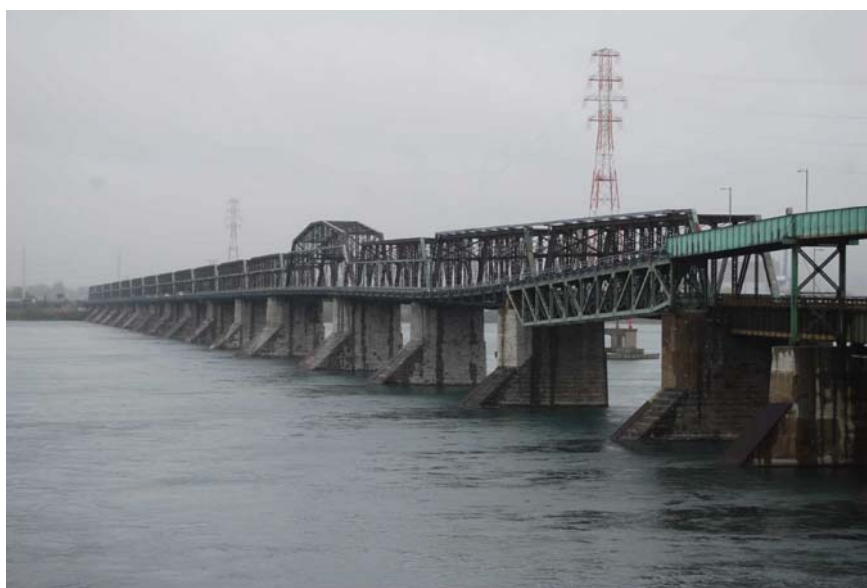
General View of Victoria Bridge and St Lawrence Seaway
