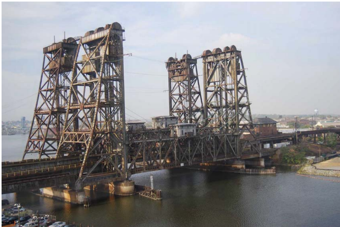
Typical NJT Lifting Bridge over the Passaic River, Newark, New Jersey
