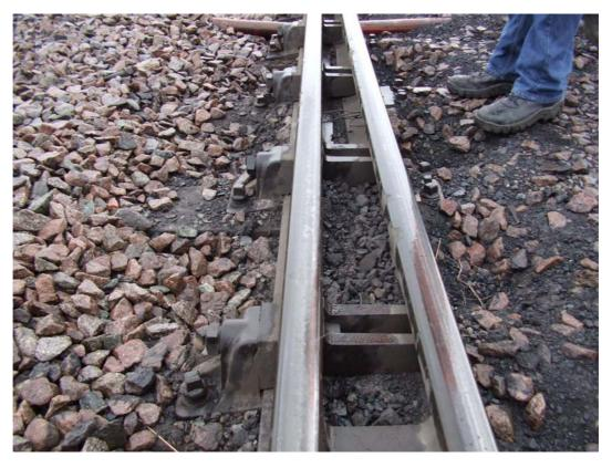
Above: Coal Spillage in moveable Switch Rail heel end Below: Severe Coal Spillage
