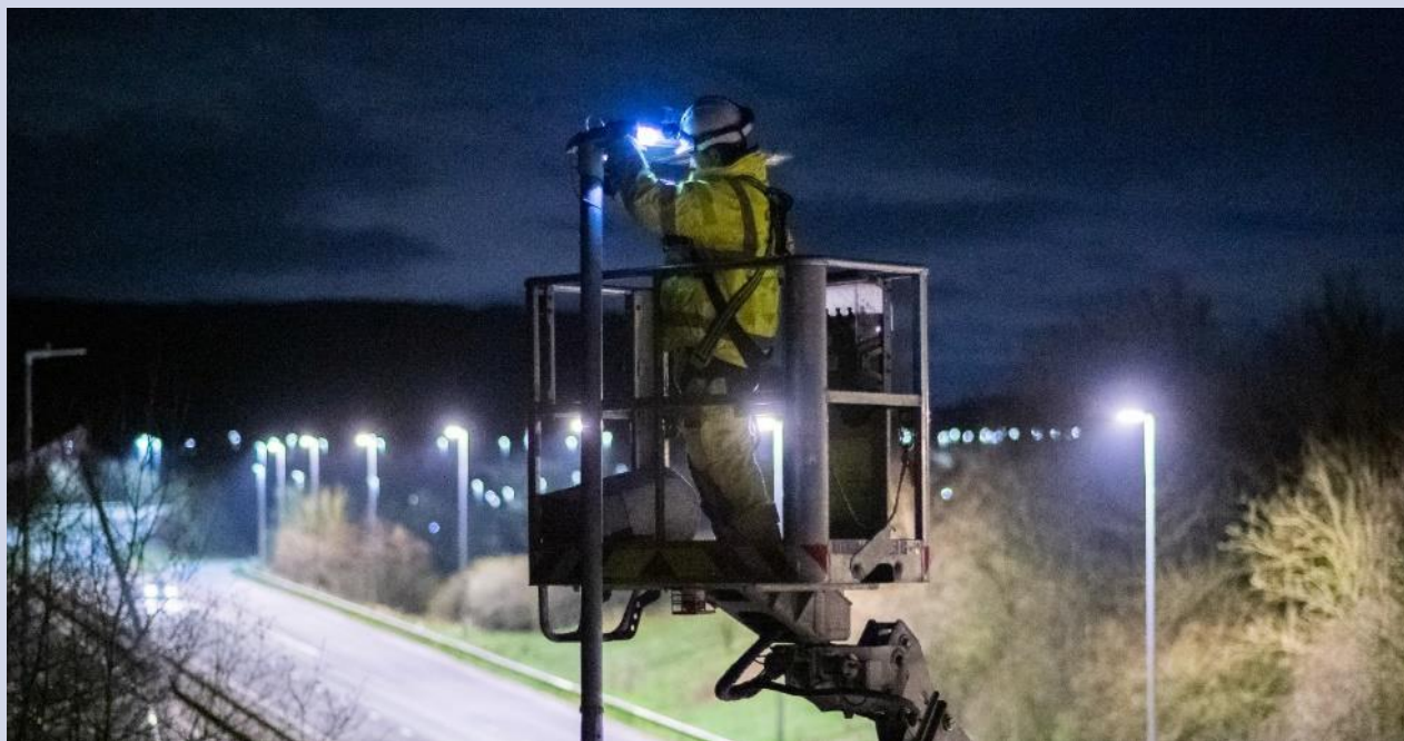
Source: National Highways, worker installing an LED bulb
