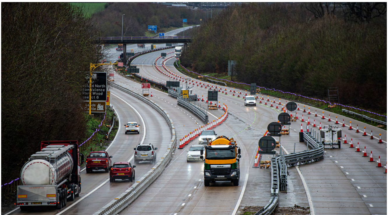
Image courtesy of Highways England
