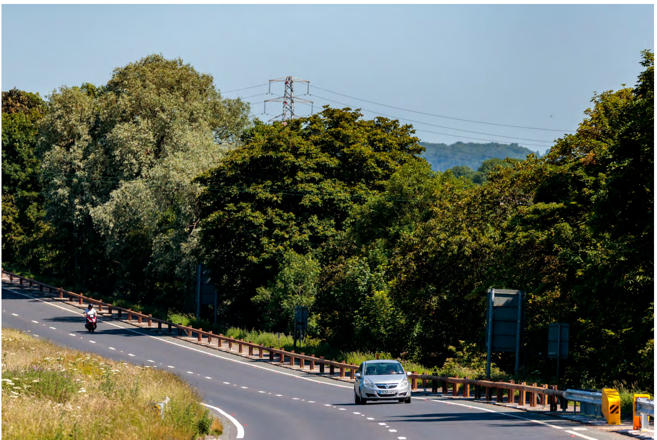
Image courtesy of Highways England
