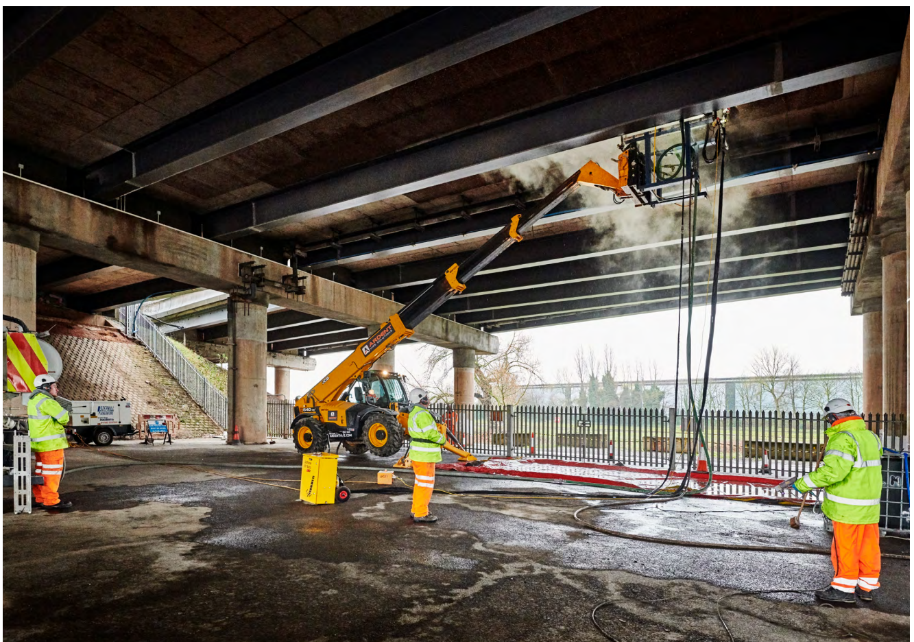
Image courtesy of Highways England
