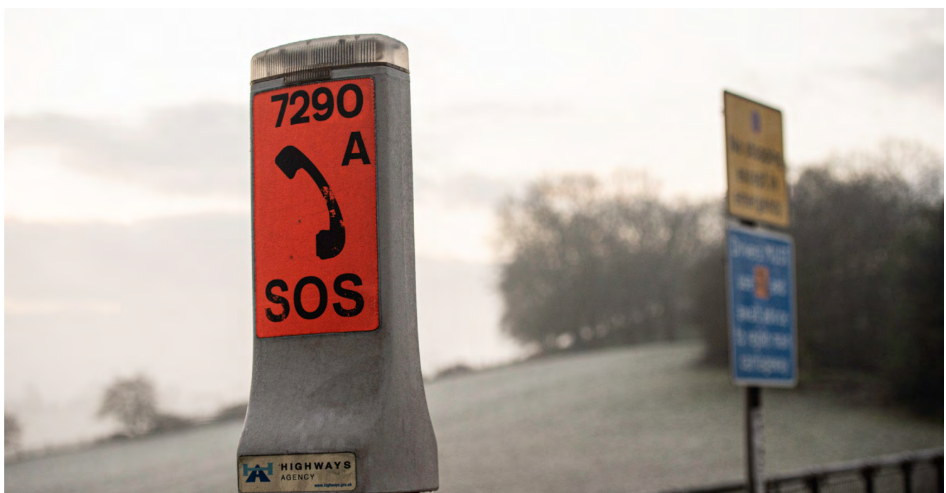
Image courtesy of Highways England
