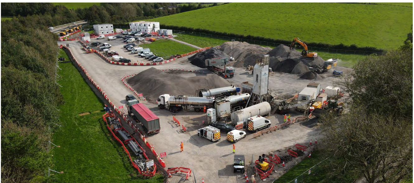
Image courtesy of Highways England
