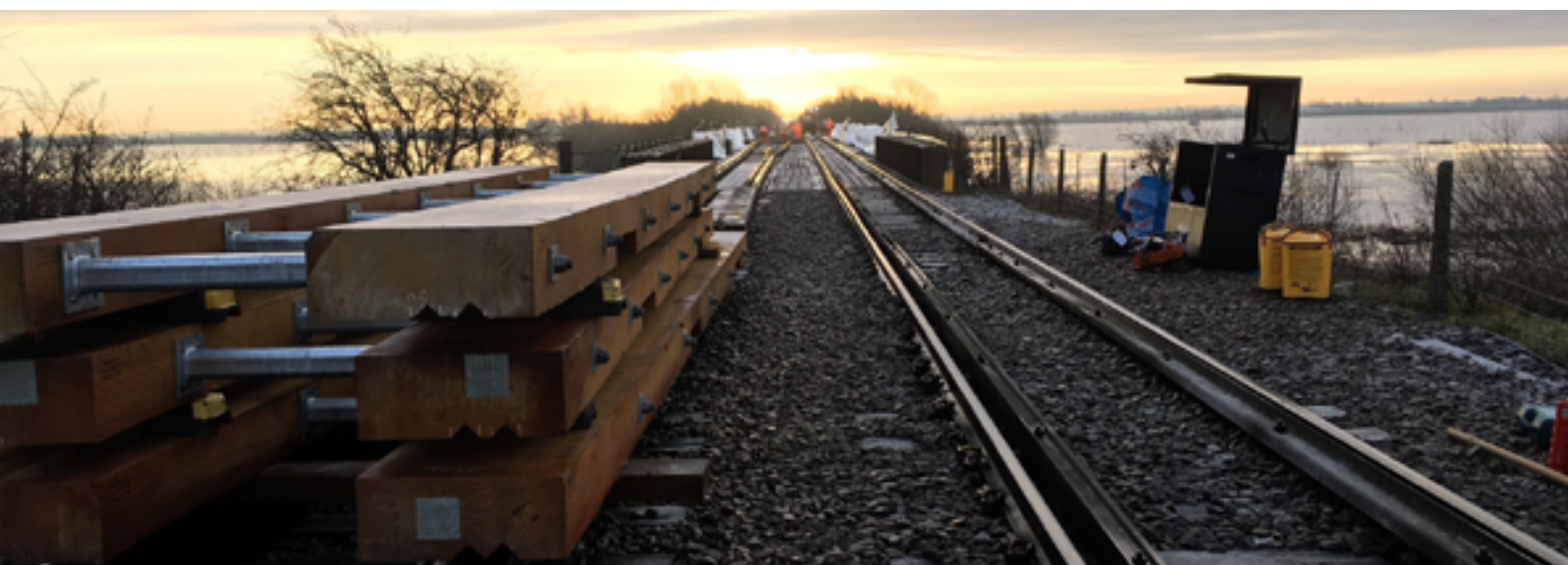
Manea Bridge, Anglia route.
