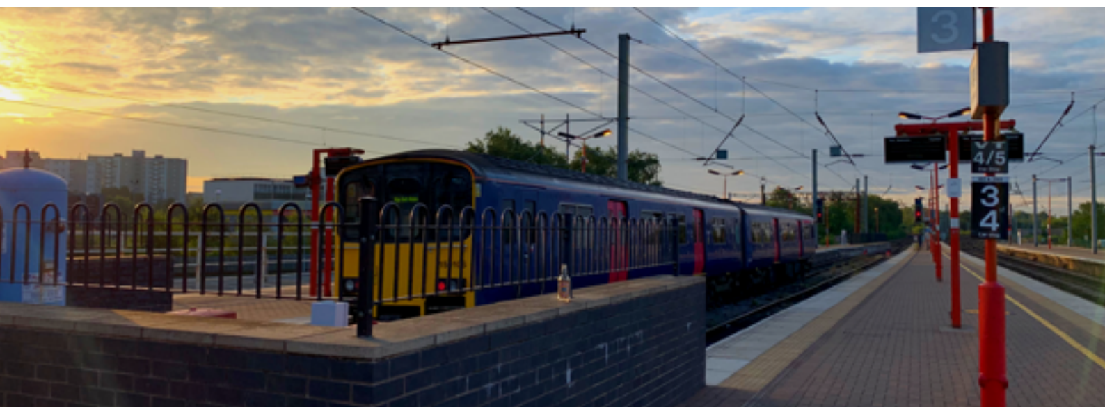
Wigan North Western Platform extension
