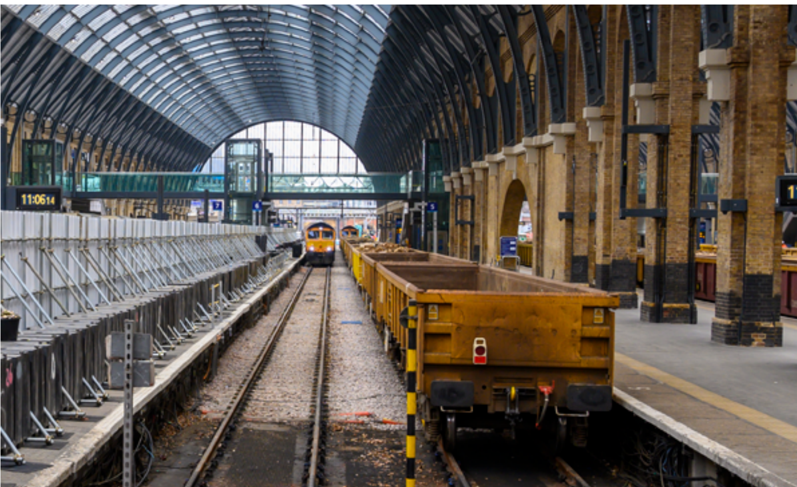
Engineering work at King's Cross station
