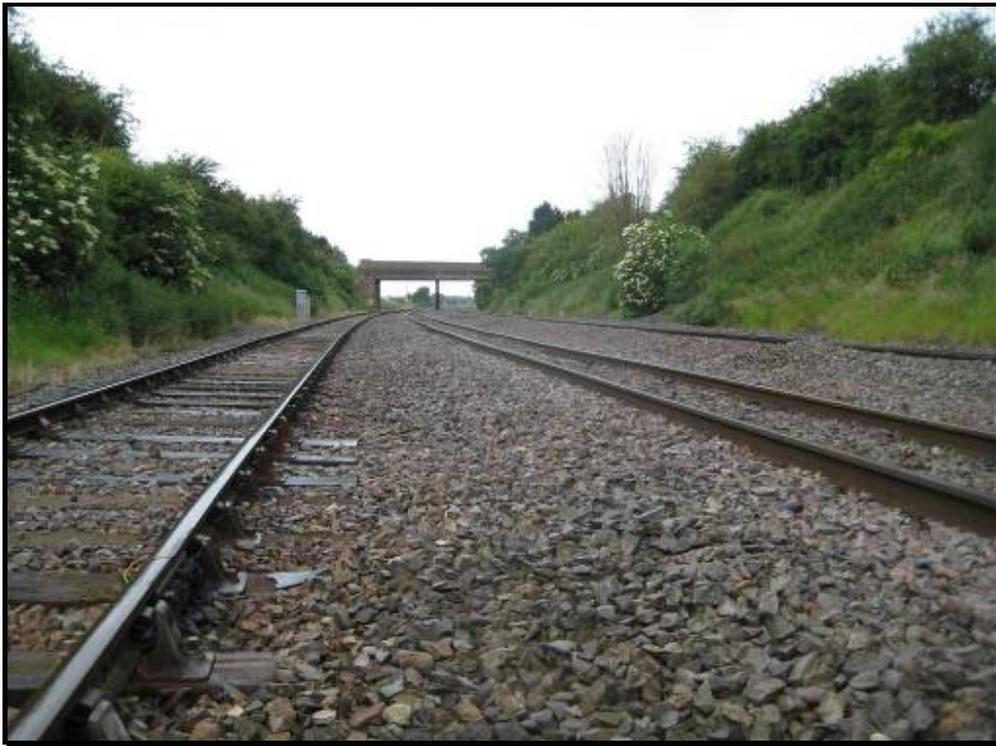
**Figure 45. Crawfords Down line looking south showing poor top.**
