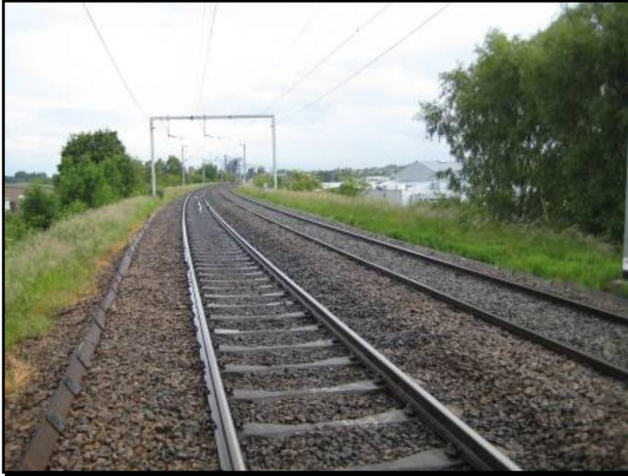
**Figure 25. View from the down line looking towards Bushbury viaduct. Note old rails in both cesses from maintenance rerailing due to sidewear.**
