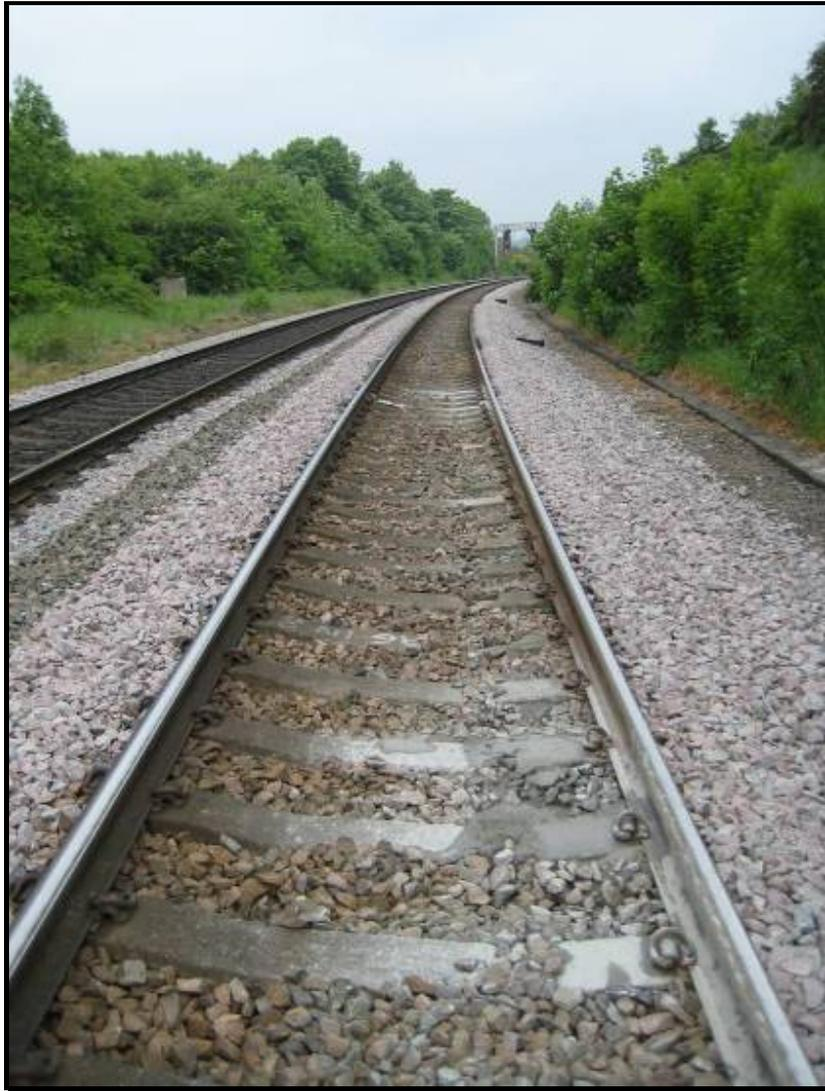
**Figure 5. The up main, south of Market Harborough, clearly showing formation failure**
