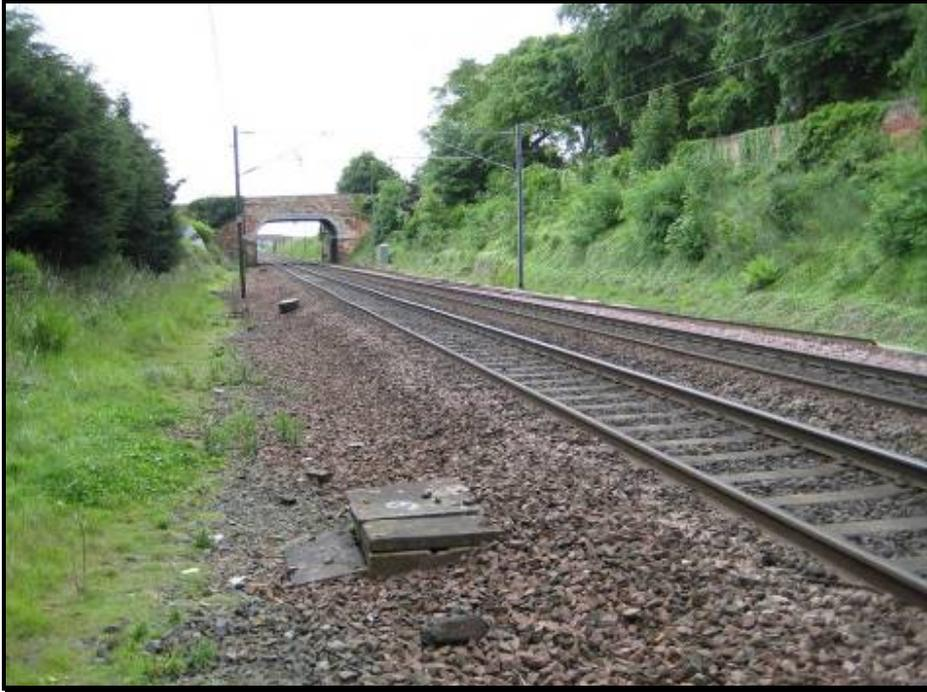
Figure 35. Monktonhall looking east through the site of the former Inveresk station, showing cess drains and poor top through overbridge 29
