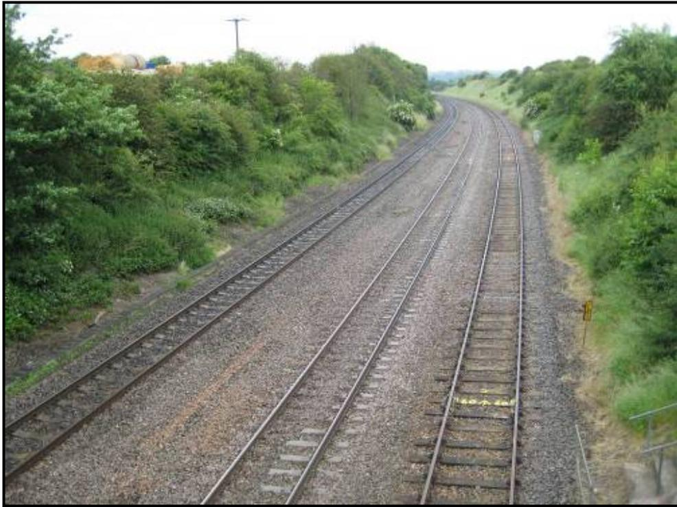
Figure 46. Picture 25. Crawfords from the overbridge looking north. Note the new cwr in the foreground and the drainage in the ten foot.
