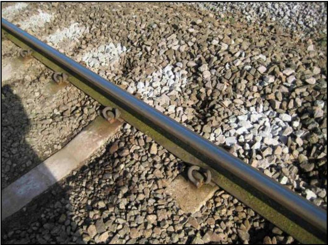
**Figure 12. Down line Barham showing the problem with slag ballast used by BR in the 1960's**
