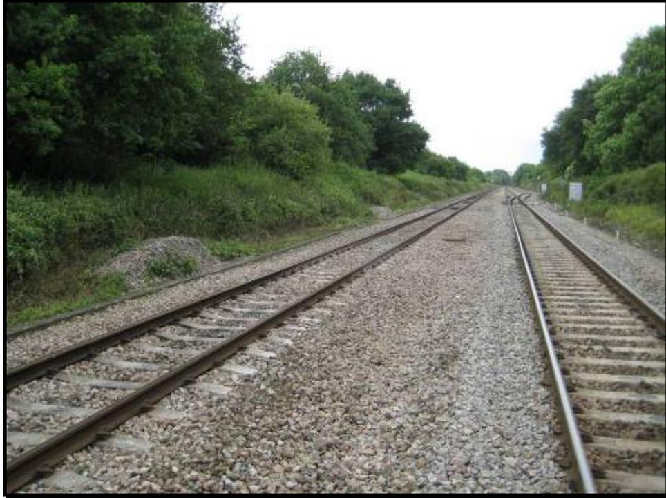
**Figure 47. Picture 26. Prouts Bridge up line from 99m 580y towards 99m 220y showing poor top and evidence of manual removal of slurried ballast.**
