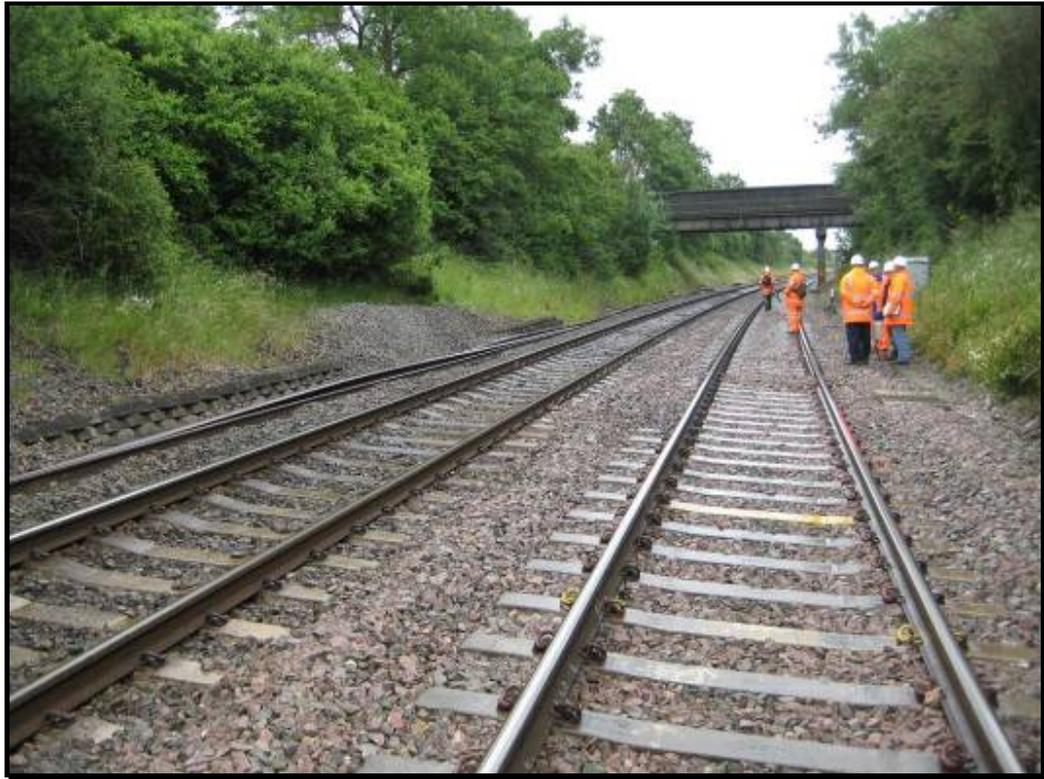
**Figure 44. Defford. View of the down line from the up showing evidence of manual repairs to the slurried ballast where the drainage system has broken down.**
