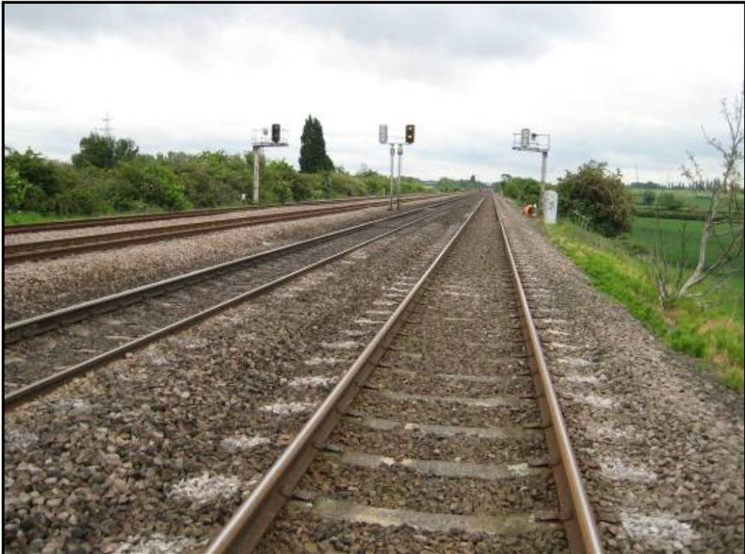
**Figure 10. Down Main at Clapham. Note voided sleepers, indicative of extending machine maintenance intervals too far.**
