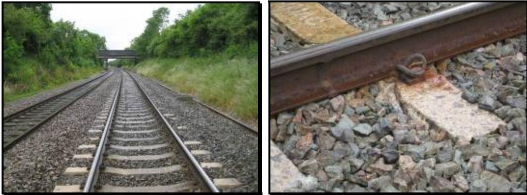
**Figures 46 and 47. Defford down line looking north (21) and damaged concrete sleepers from a derailment many years ago (22). The formation problems are in the vicinity of the overbridge.**
