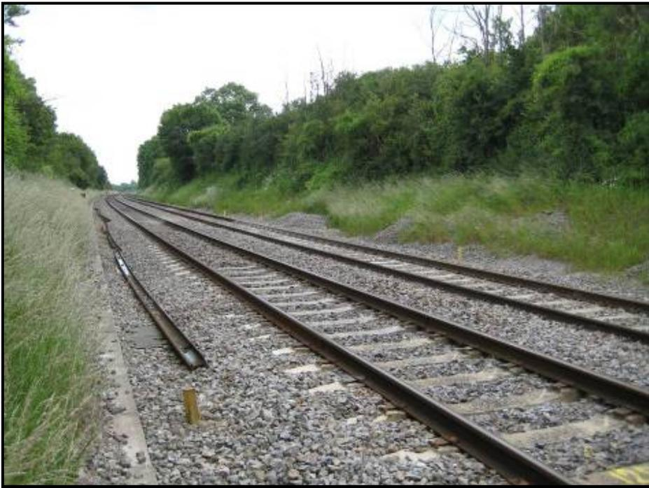
**Figure 48. Both tracks are proposed for renewal. The up line is in the foreground. Note the evidence of manual treatment to the slurried ballast on the down.**
