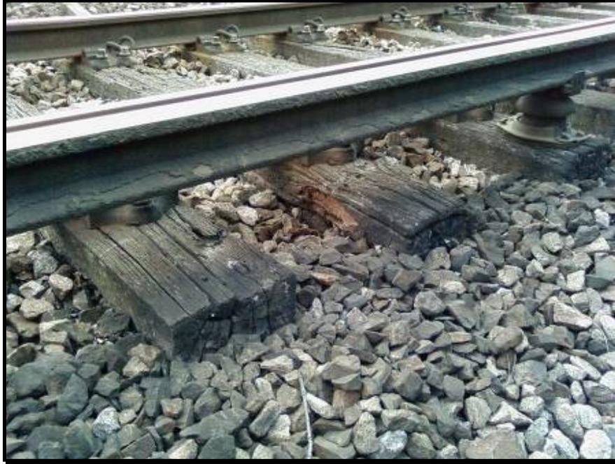
Figure 18. General sleeper condition at Surbiton is very poor.
