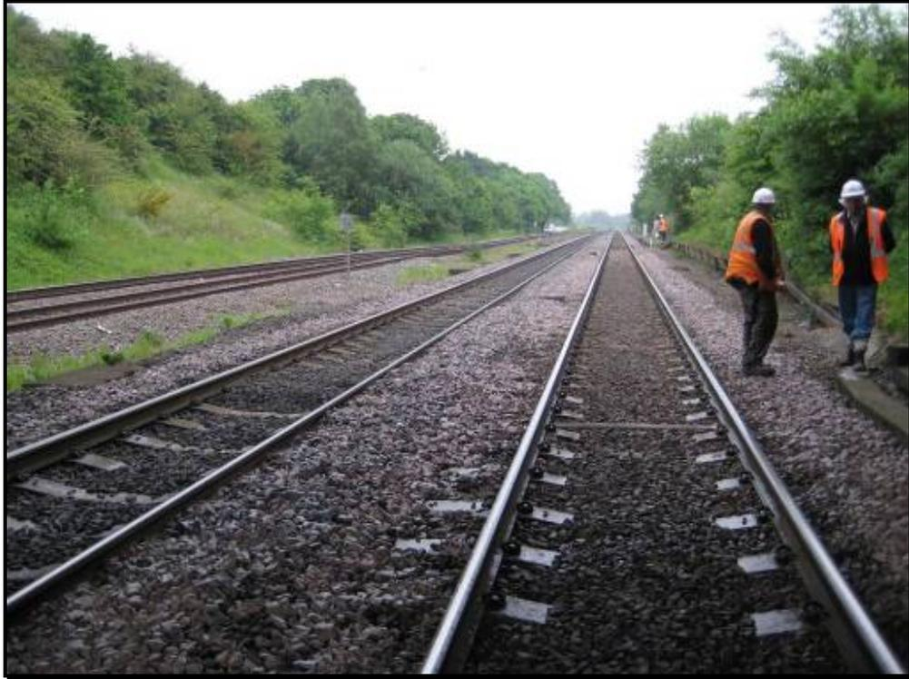
**Figure 7. Kettering. View looking south towards Kettering South Junction. Note the existing drainage manholes in the up cess, six foot and down cess.**
