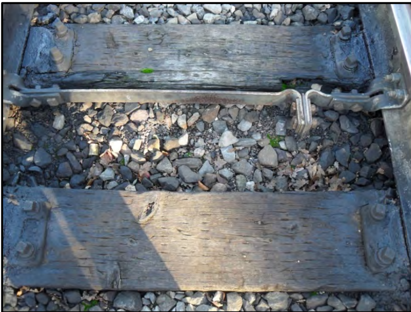
Figure 5-7 Replacement timbers in 5A Pts
