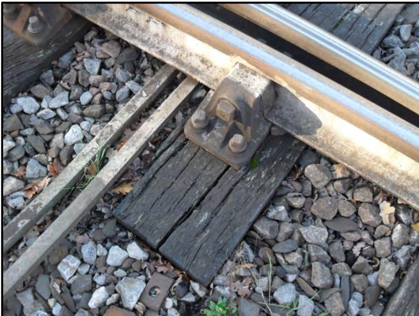
Figure 5-9 Typical Original timber bearer in single turnout 4A pts
