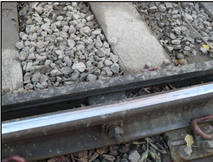
Figure 5-20 Worn Check rail
