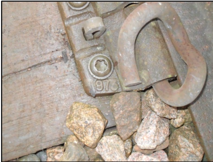
Figure 5-25 Pan 8 baseplate with Titgermeyer screw
