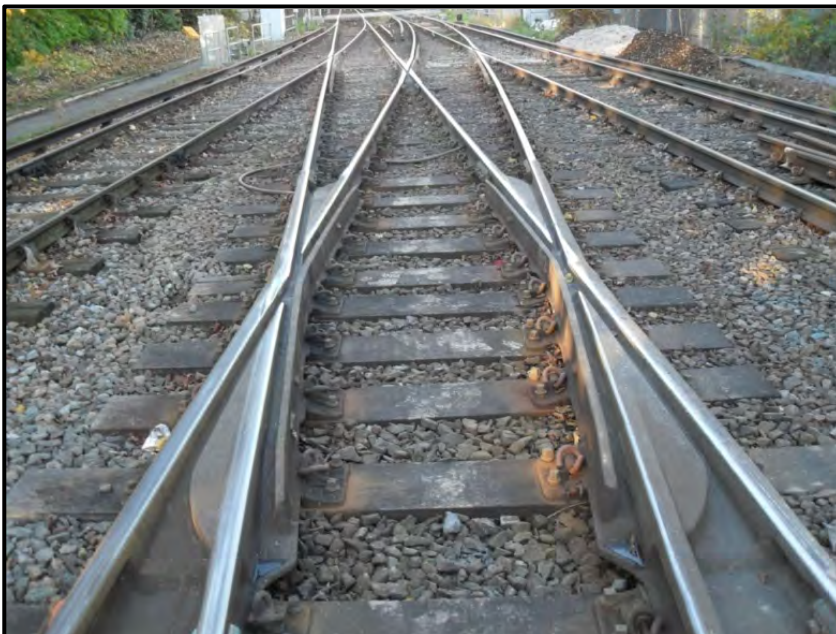
Figure 5-12 Re-timbering under diamond
