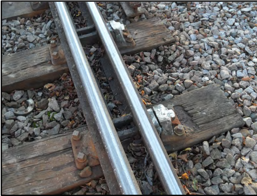
Figure 5-19 Loose Jaw Blocks
