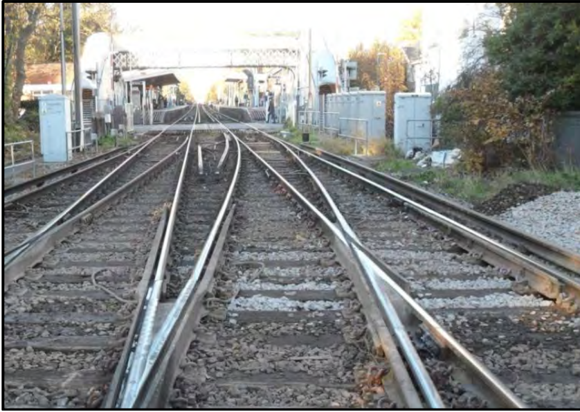
Figure 5-15 Reballasting under common crossing
