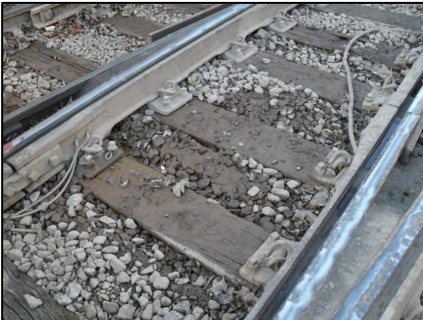
Figure 5-14 Wet bed area under crossings
