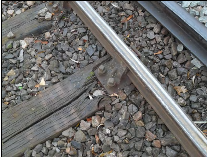
Figure 5-22 Split timber and chair indentation
