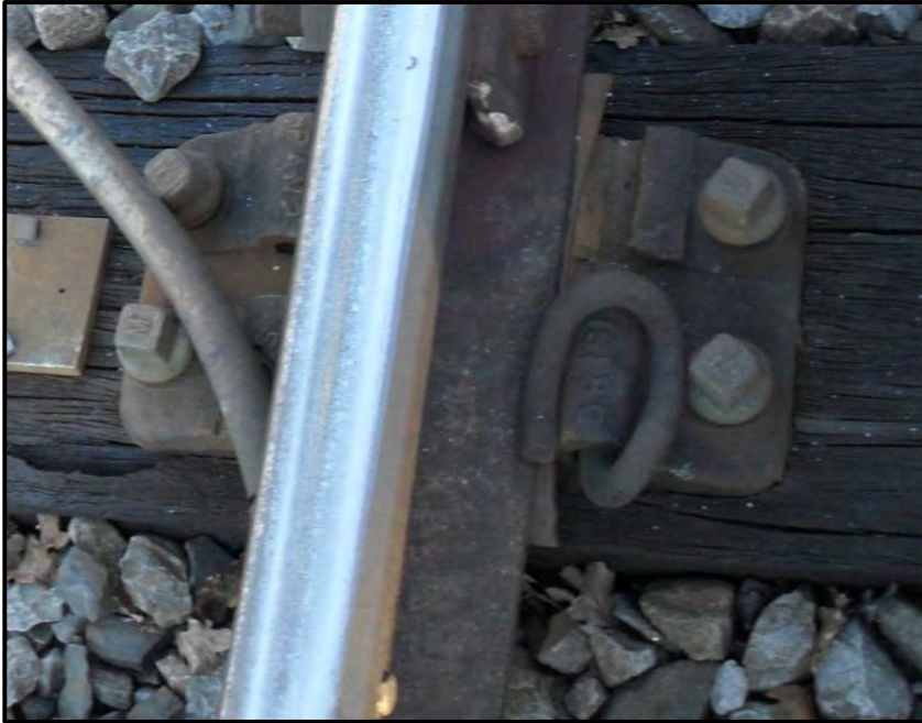
Figure 5-8 Maintenance coach screws
