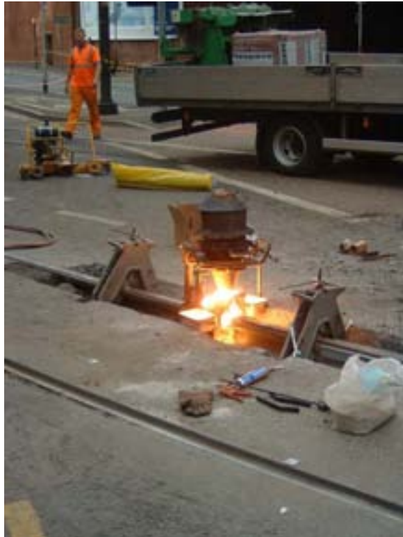
(a) Welding a rail joint
