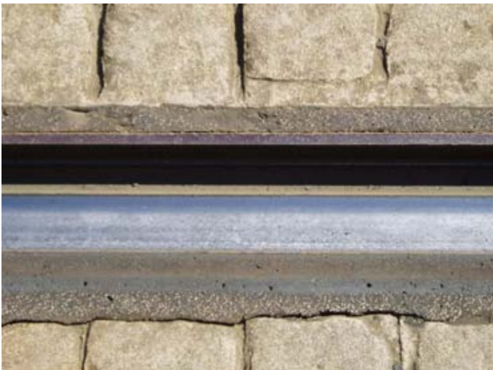
FES0409-01/81 (b) Grooved rail near the Cathedral tram stop (07.09.04)
