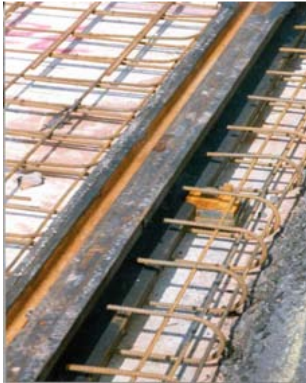
Figure 6.2 Midland Metro grooved rail track during construction
