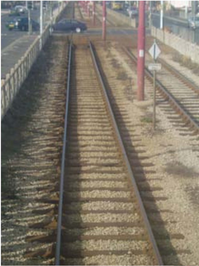
(a) Ballasted track and level crossing
