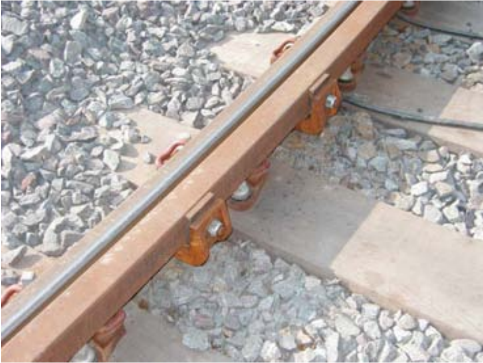
Figure 8.17 Check rail fitted to Depot curved track
