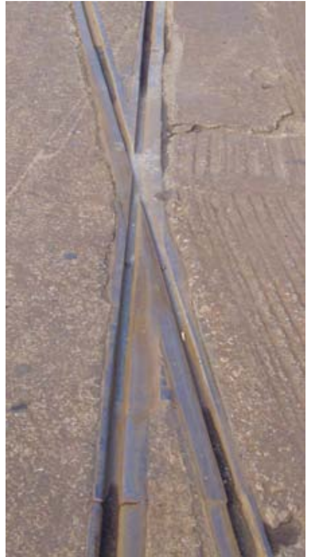
(b) Flange tip running crossing
