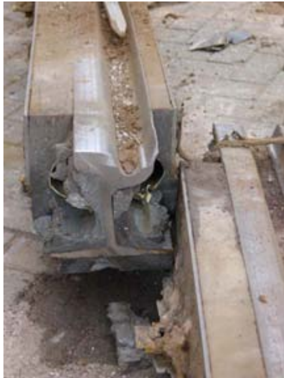
(a) Rail removed from concrete channel
