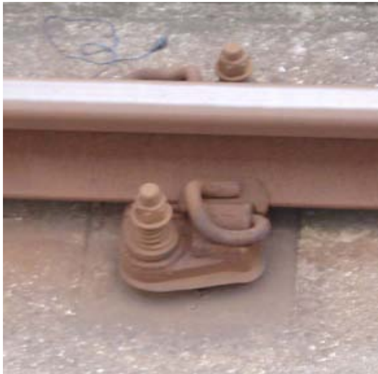
Figure 4.11 Slab track resilient rail fastening on the Docklands Light Railway (22.10.04)
