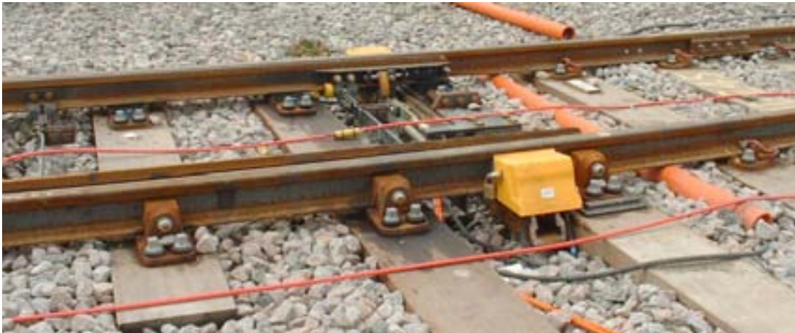
Figure 4.24 Ballasted track turnout linking the Beckton Up line to the City Airport extension of the Docklands Light Railway
