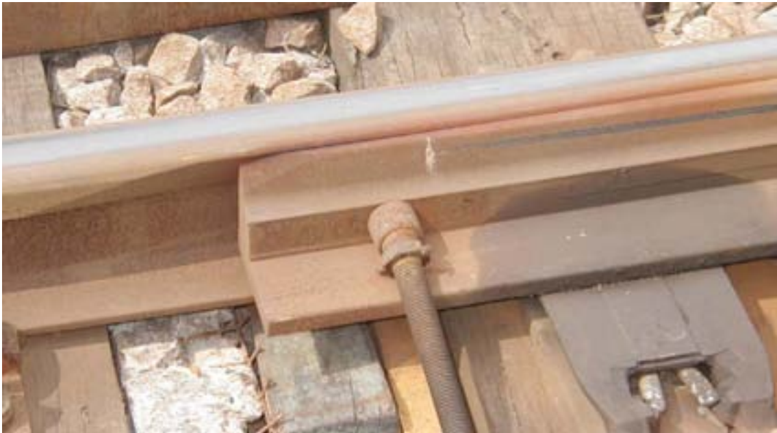
(a) Blade tip in good condition (07.08.02) at Elmers End
