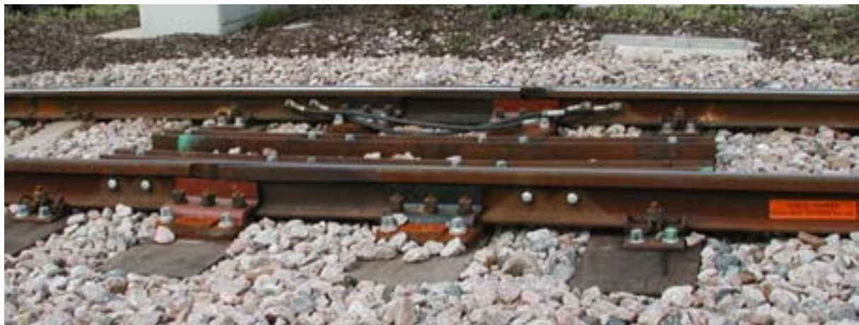
Figure 3.12 Ballasted track expansion switch (07.08.02), Croydon Tramlink
