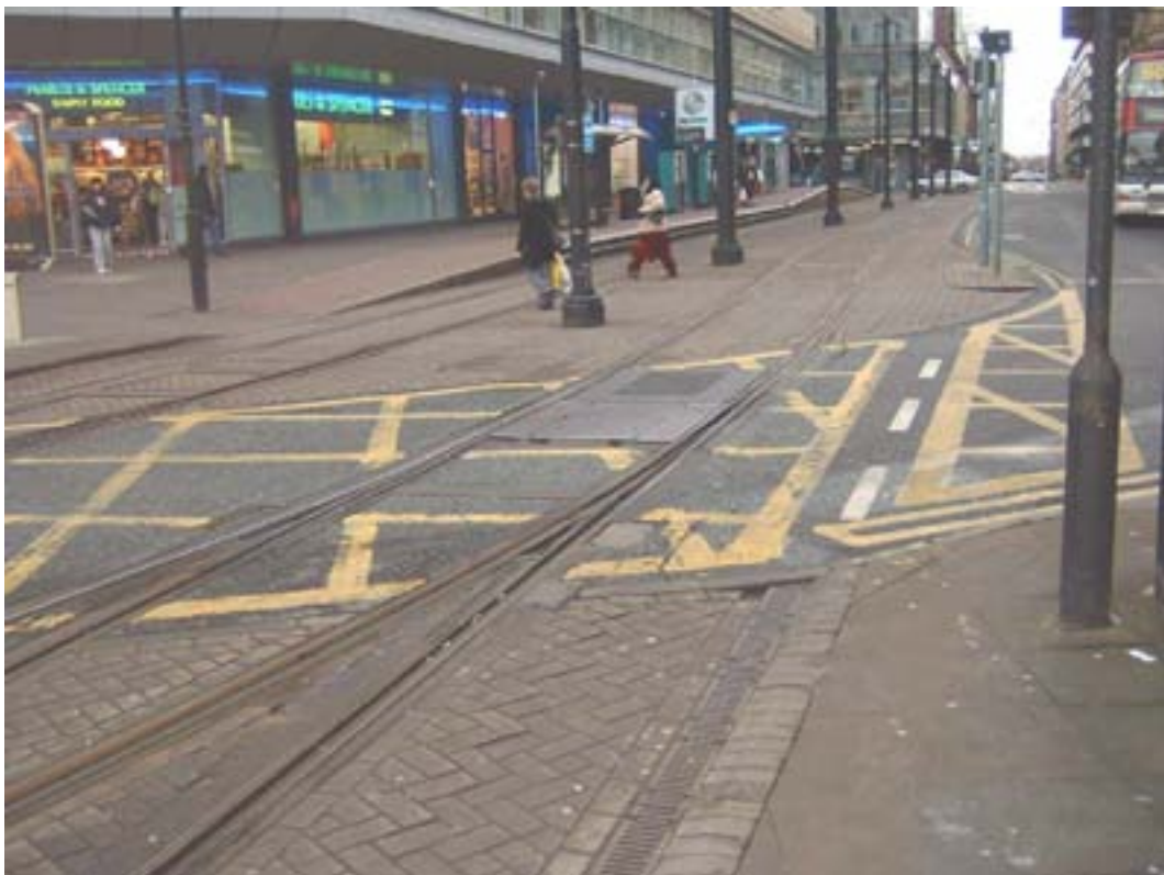
Figure 5.11 Bus lane crossing a turnout on Mosley Street, Manchester Metrolink
