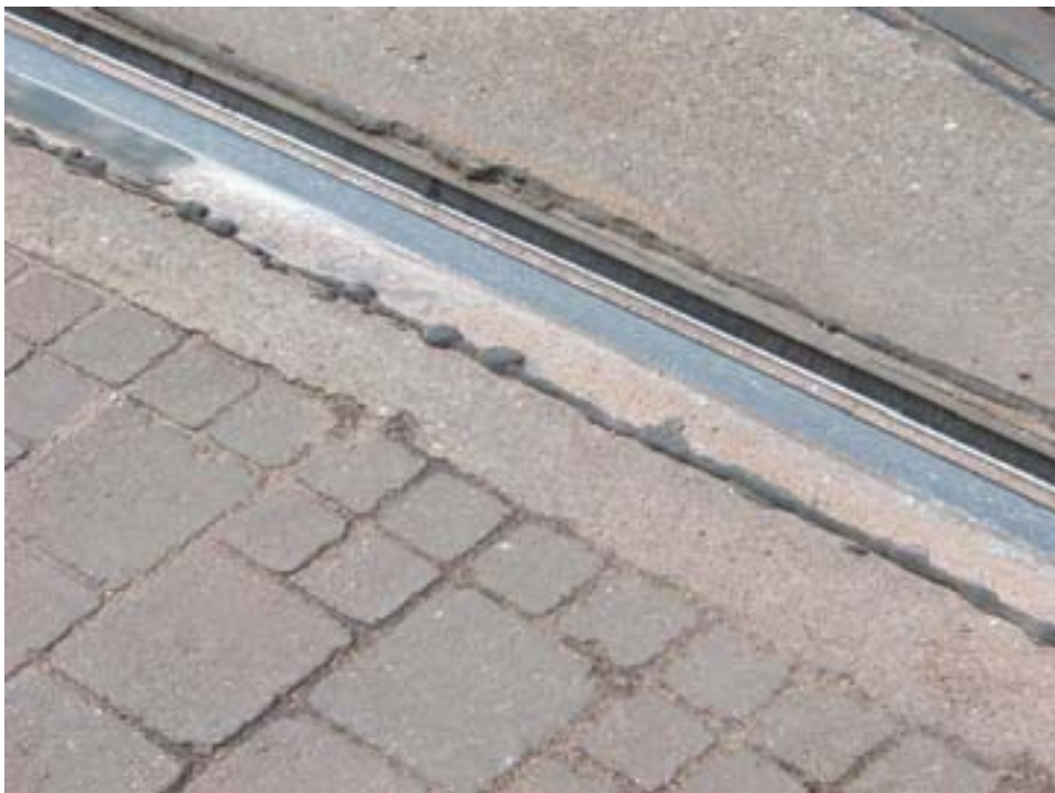
Figure 6.3 Midland Metro grooved rail keeper flange wear at Wolverhampton St Georges (11.06.02)
