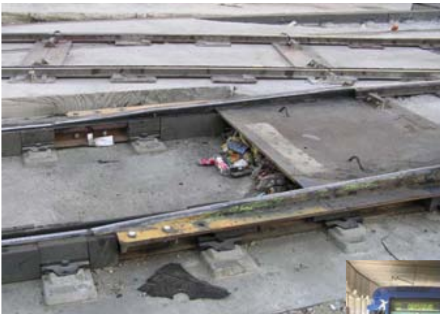
(b) Detail of 'ramp' rails
