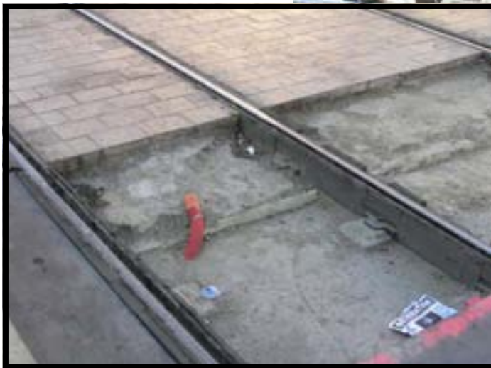
(b) View showing installation of brick surfacing
