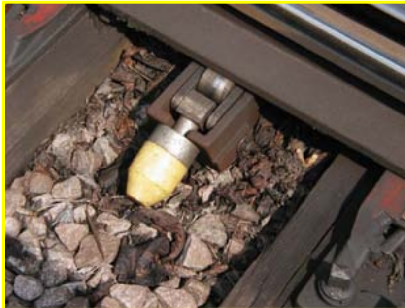
(b) Detail of a Schreck-Mieves roller support
