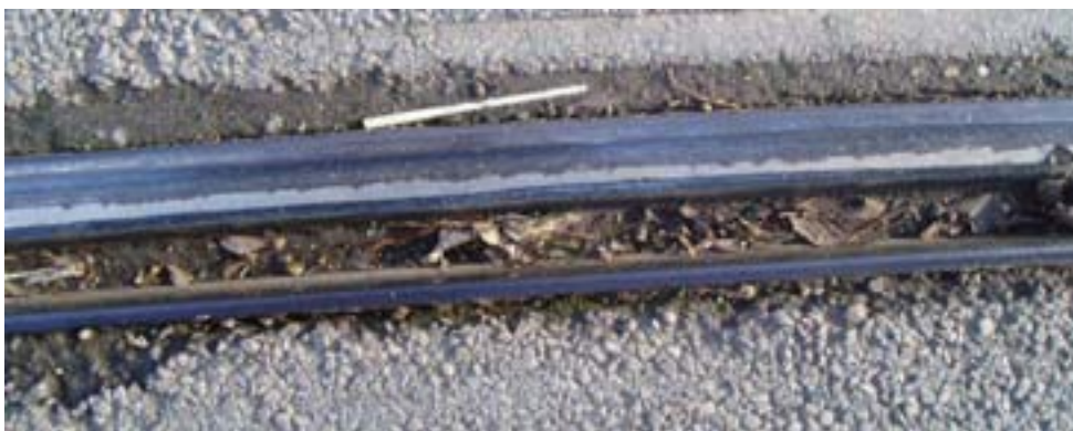
FES0410-01/42 (d) Wheel wear mark on rail head at Fleetwood Ferry
