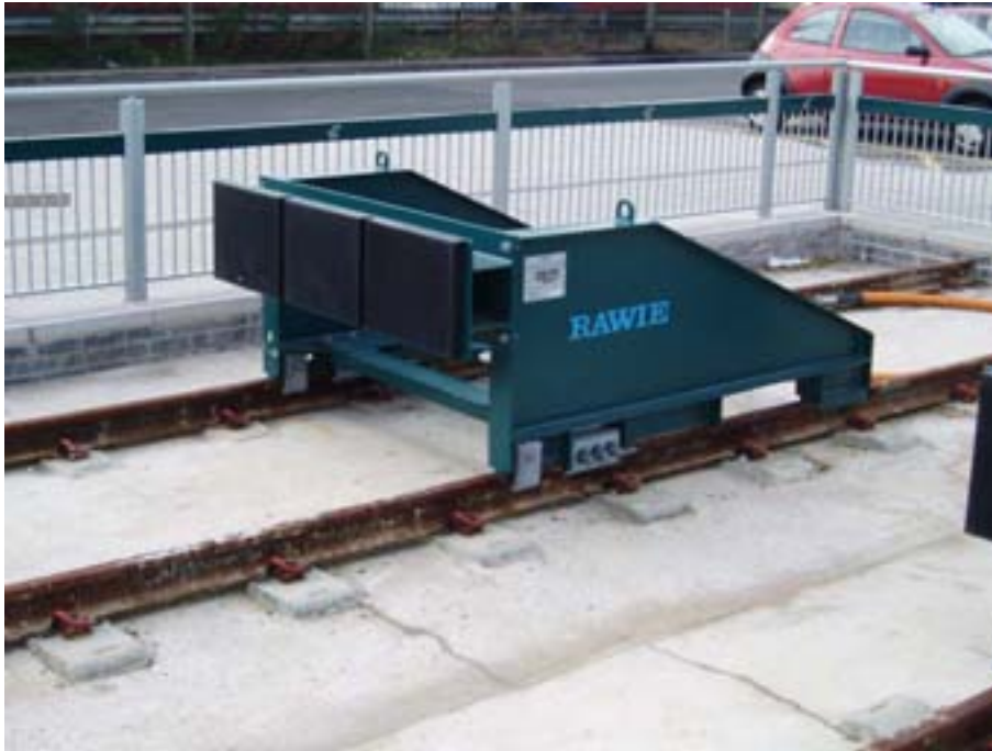
Figure 8.13 Buffer unit on concrete embedded sleeper track at the Hucknall terminus (11.09.04)
