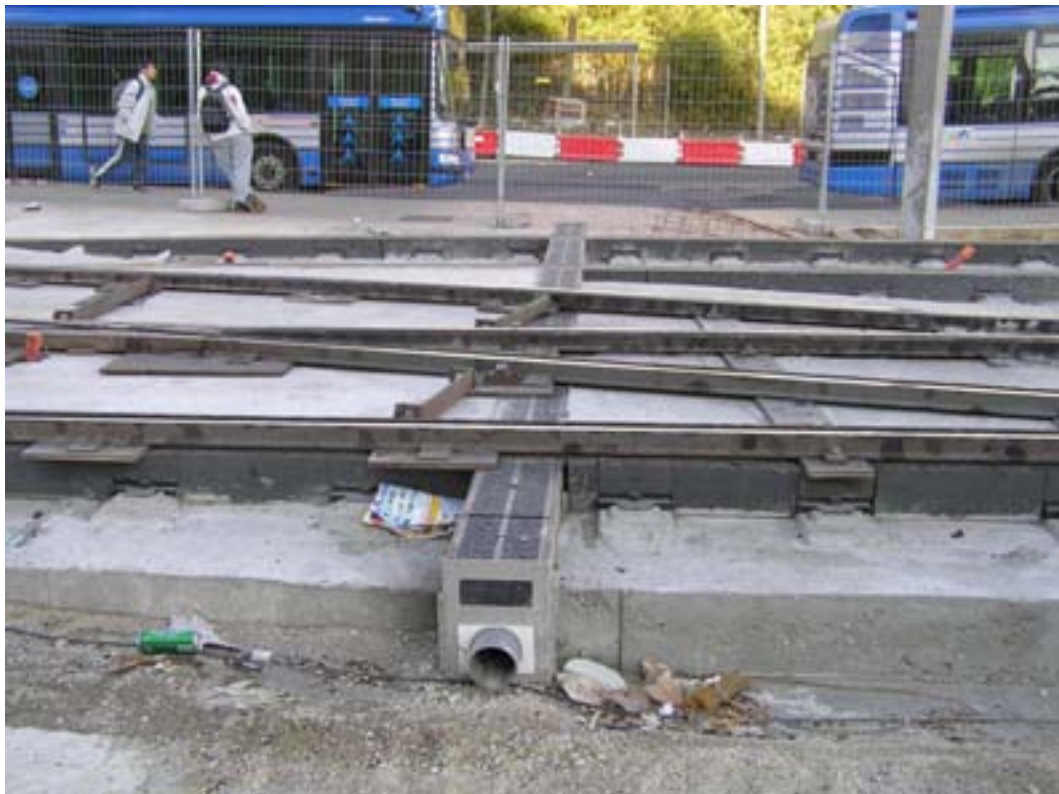
Figure 11.17 Method of track drainage, TaM Montpellier (03.03.05)
