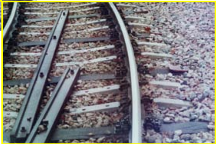
Figure 3.10 Bracing fitted to ballasted track, Croydon Tramlink
