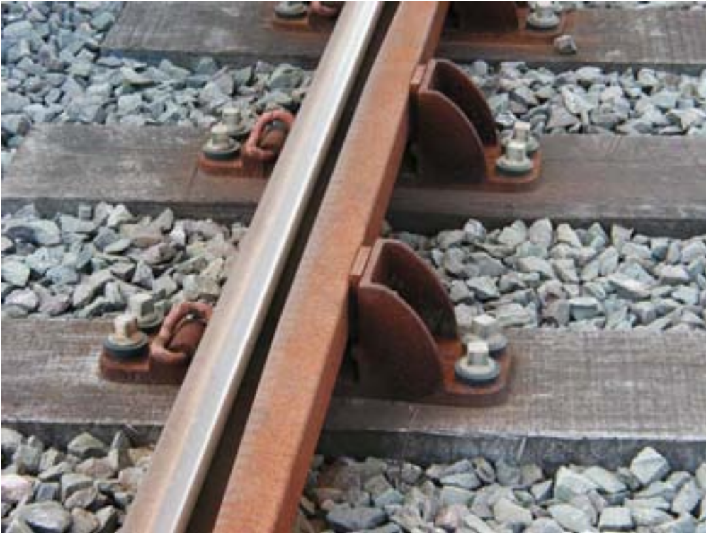
Figure 6.9 Midland Metro adjustable check rail with spacers associated with 100m radius turnout
