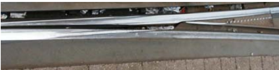
(b) Switch rail at East Croydon
