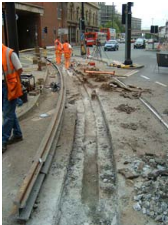
(b) New polymer coated rail ready for installation
