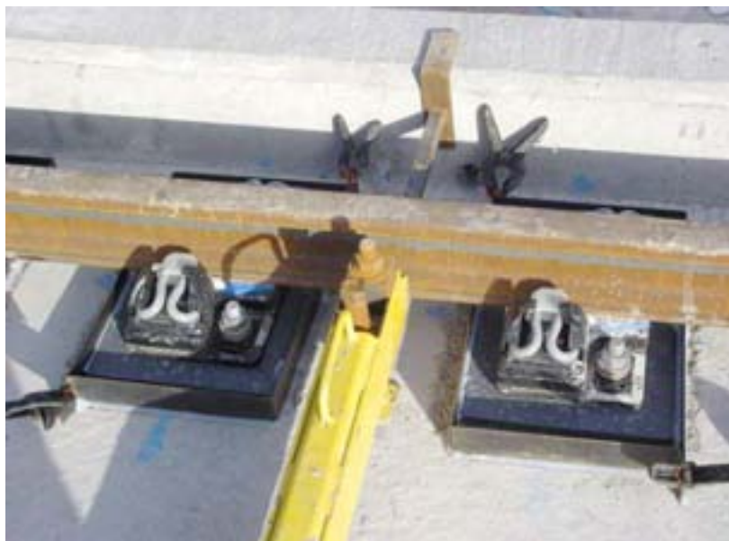
(c) Formwork around baseplates prior to pouring grout
