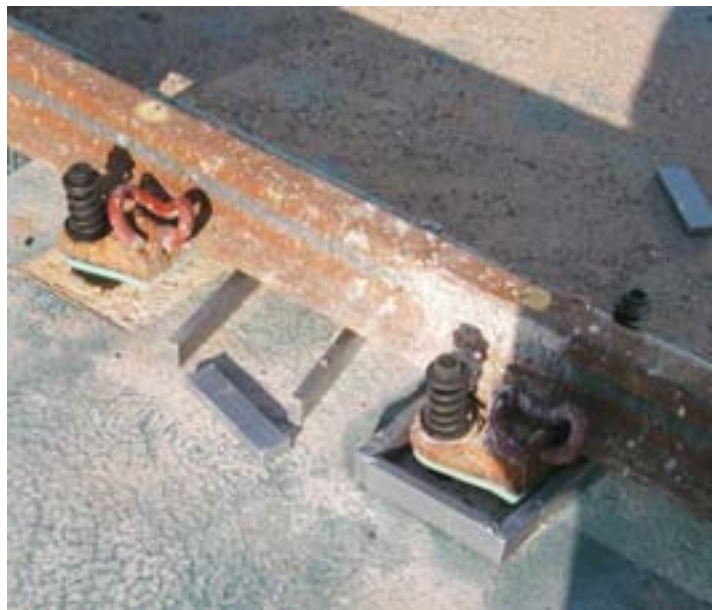
Figure 8.9 Completed NET grooved rail track, 18m radius curve (05.02.02)
