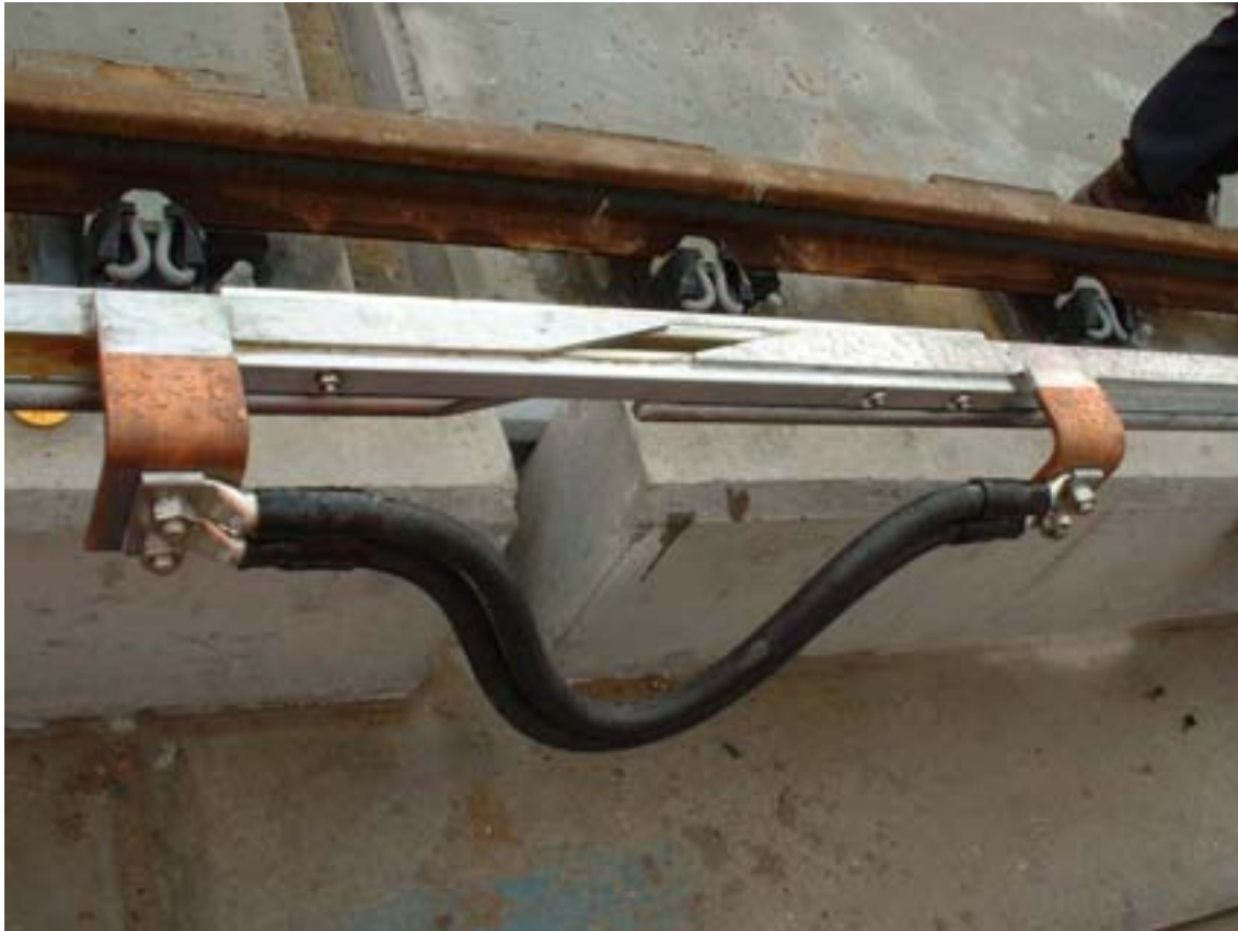
Figure 4.27 Conductor rail expansion joint prior to installation of the protective shroud, City Airport extension of the Docklands Light Railway
