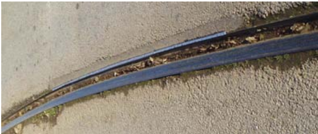
FES0410-01/38 (c) Repair to keeper flange, Fleetwood Ferry
