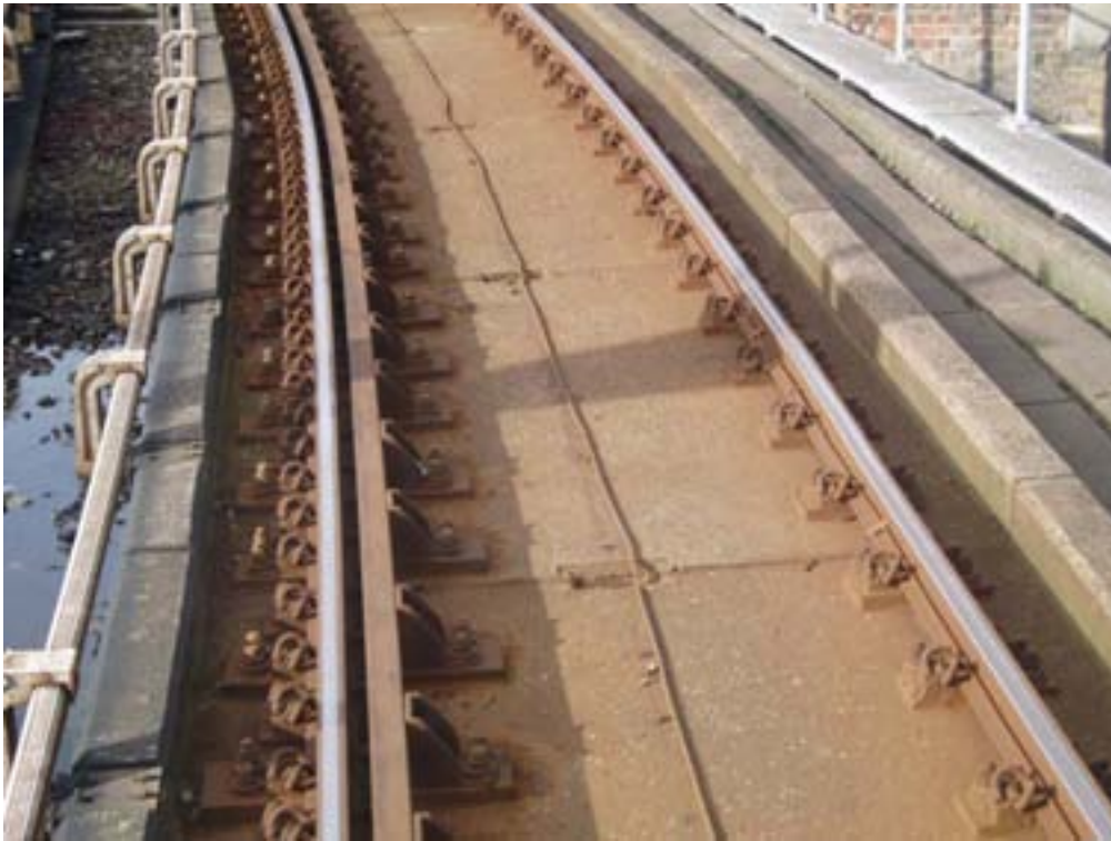
Figure 4.8 Slab track plain line and guard rail resilient fastenings on the Docklands Light Railway (22.10.04)
