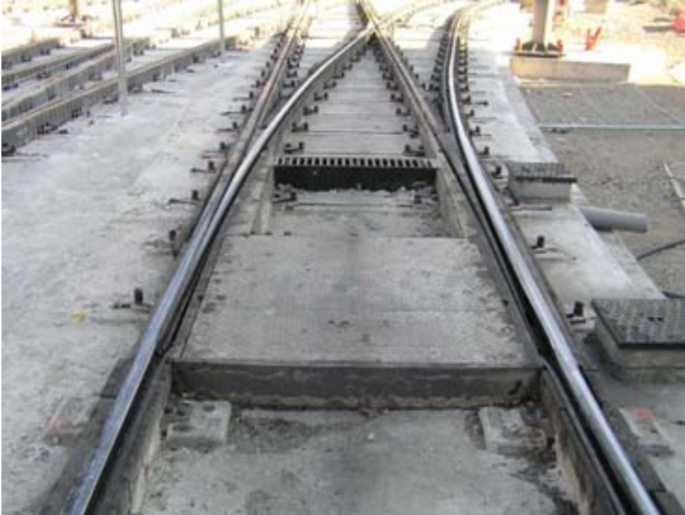
(a) Turnout during construction
