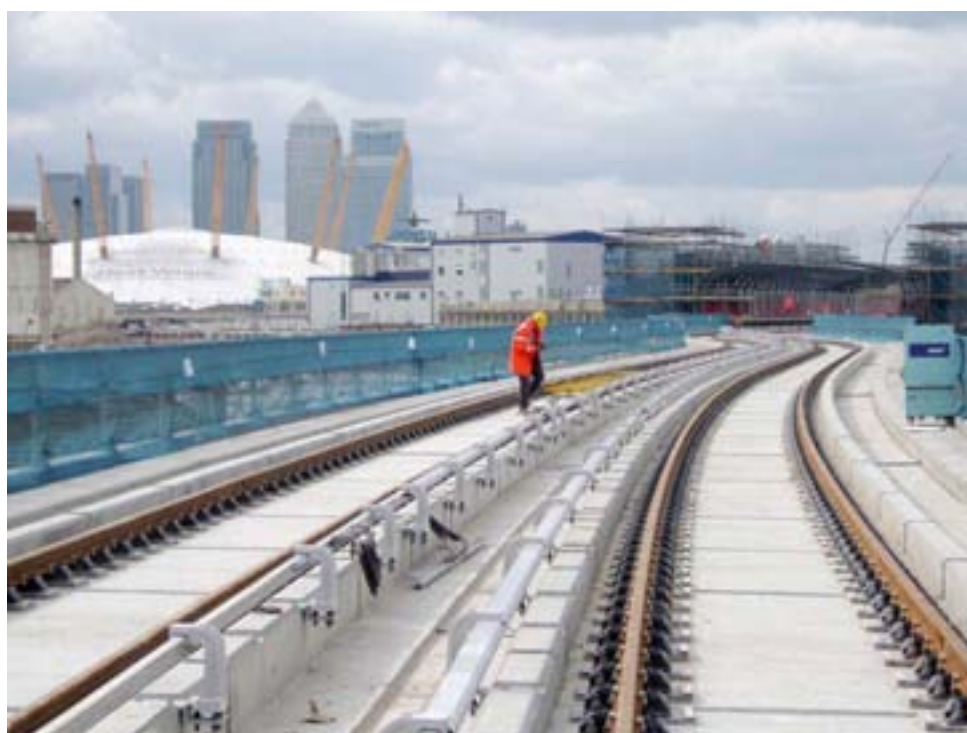
Photo courtesy of Pandrol UK Ltd (b) Baseplate grouting completed
