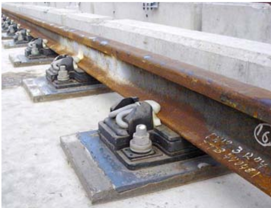
Photo courtesy of Pandrol UK Ltd (a) Baseplate grouting completed
