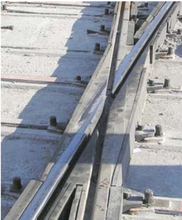
(a) Turnout during construction
