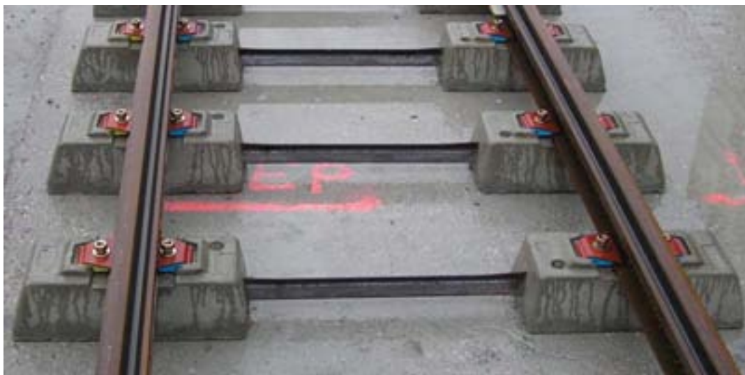
(c) Grooved rail track during assembly
