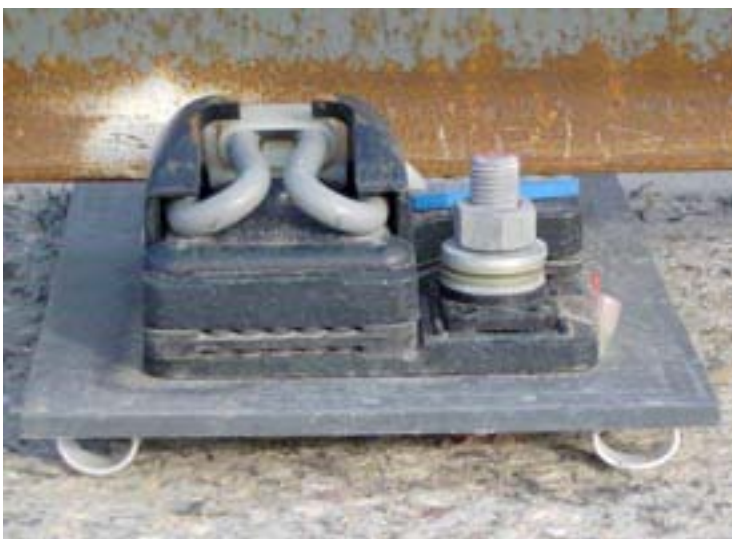
(b) Baseplate positioned for grouting
