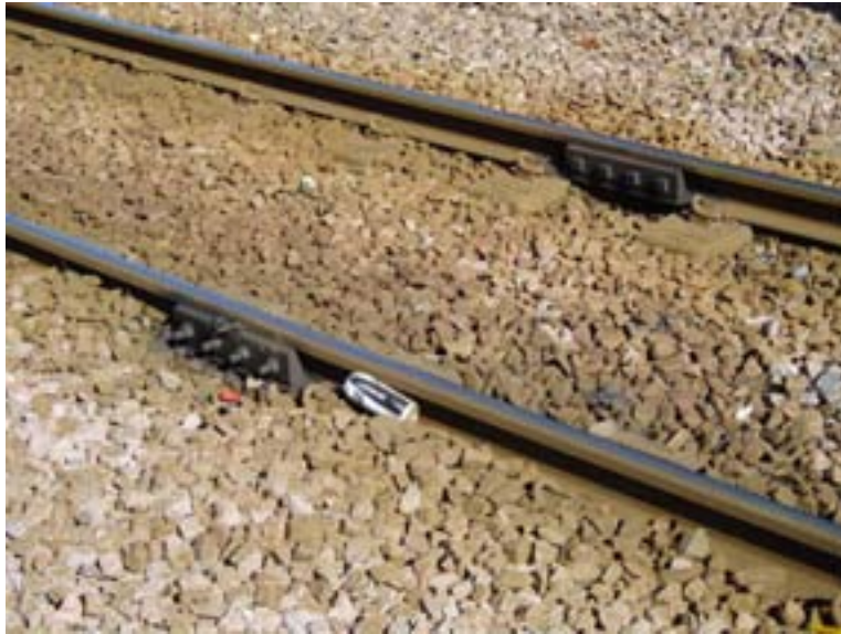
Figure 9.5 Example of SYS ballasted track with twin block sleepers (07.09.04)
