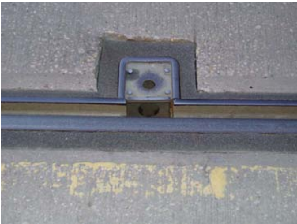
Figure 9.4 Examples of grooved rail drainage in West Street, SYS (07.09.04)
