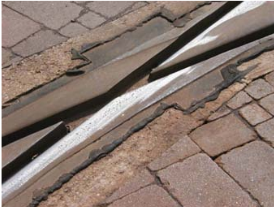
(a) Turnout crossing at Wolverhampton St Georges
