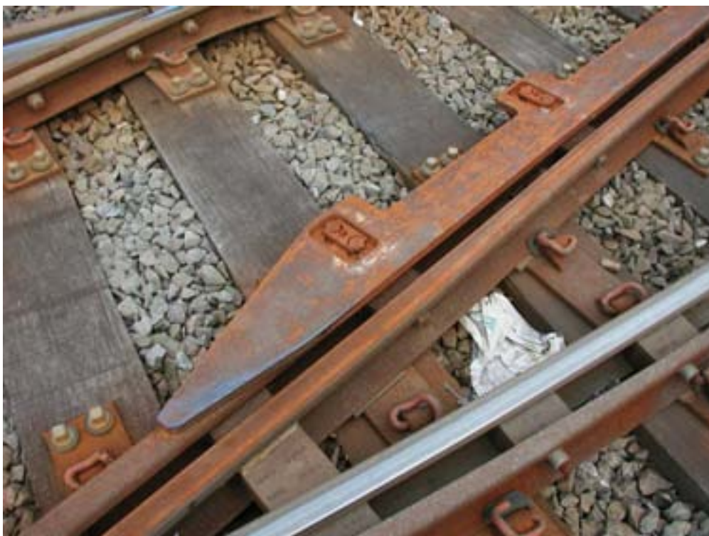
Figure 6.9 Midland Metro adjustable check rail with spacers associated with 100m radius turnout
