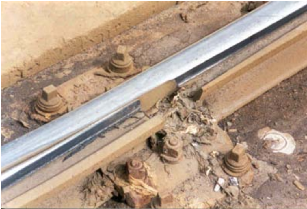
(b) Worn expansion switch
