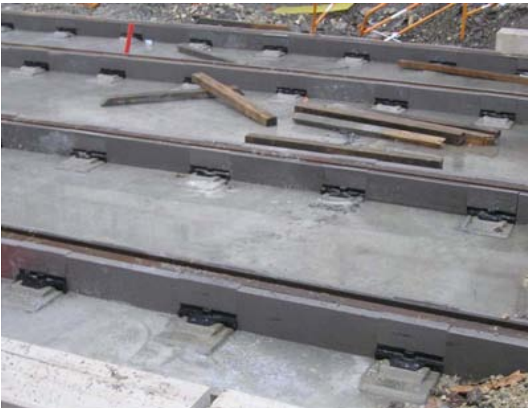
(b) Track following concreting of sleeper and with rail cladding in place
