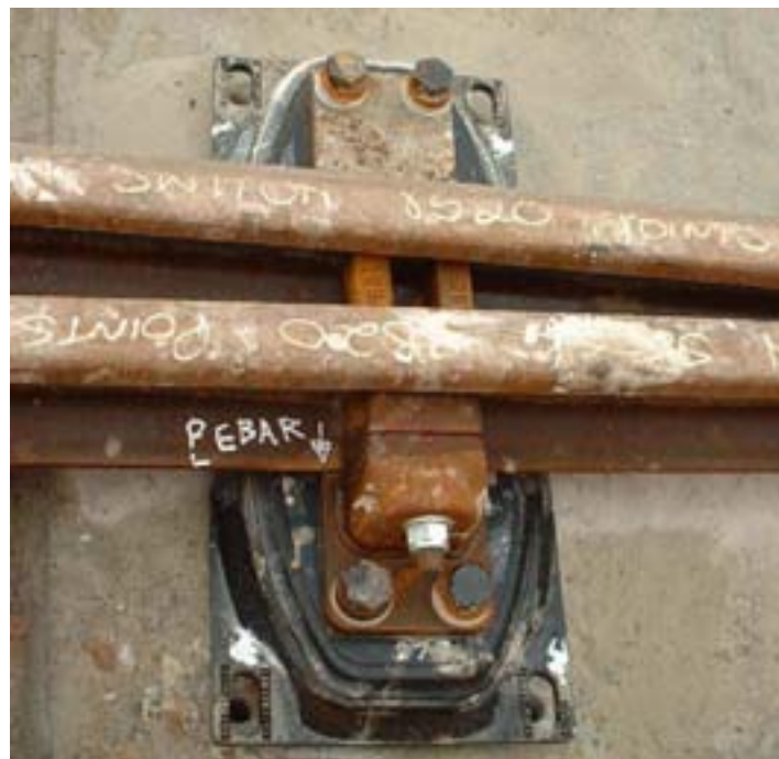
Figure 4.21 The original design of slab track swing nose turnout Docklands Light Railway
