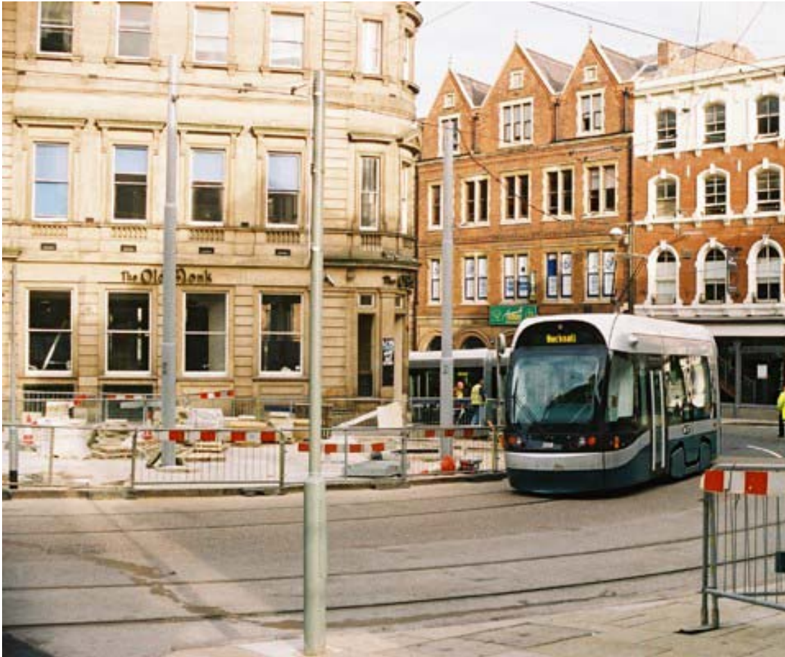
Figure 8.9 Completed NET grooved rail track, 18m radius curve (05.02.02)
