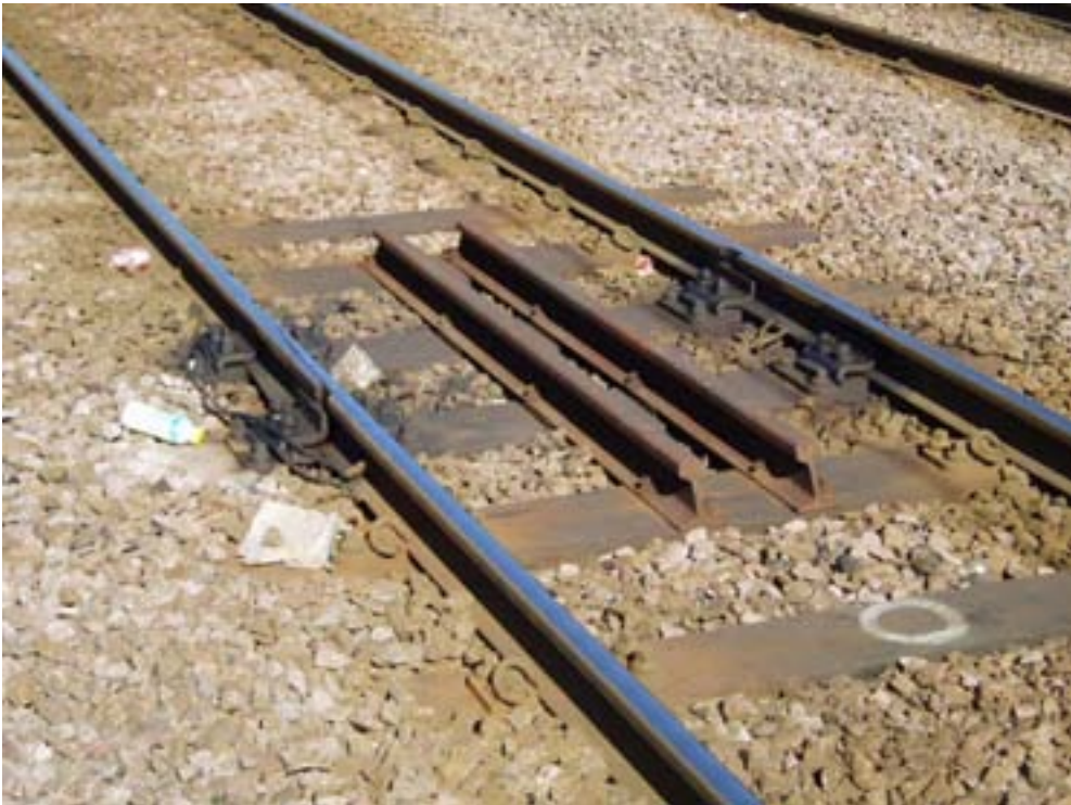
Figure 9.7 Example of a SYS expansion joint on ballasted track close to Sheffield Station tram stop (07.09.04)
