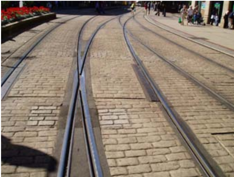
Figure 9.9 Sacrificial check rail fitted to grooved rail turnout, close to the SYS Cathedral tram stop (07.09.04)
