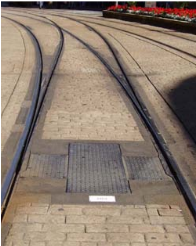
Figure 9.7 Example of a SYS expansion joint on ballasted track close to Sheffield Station tram stop (07.09.04)
