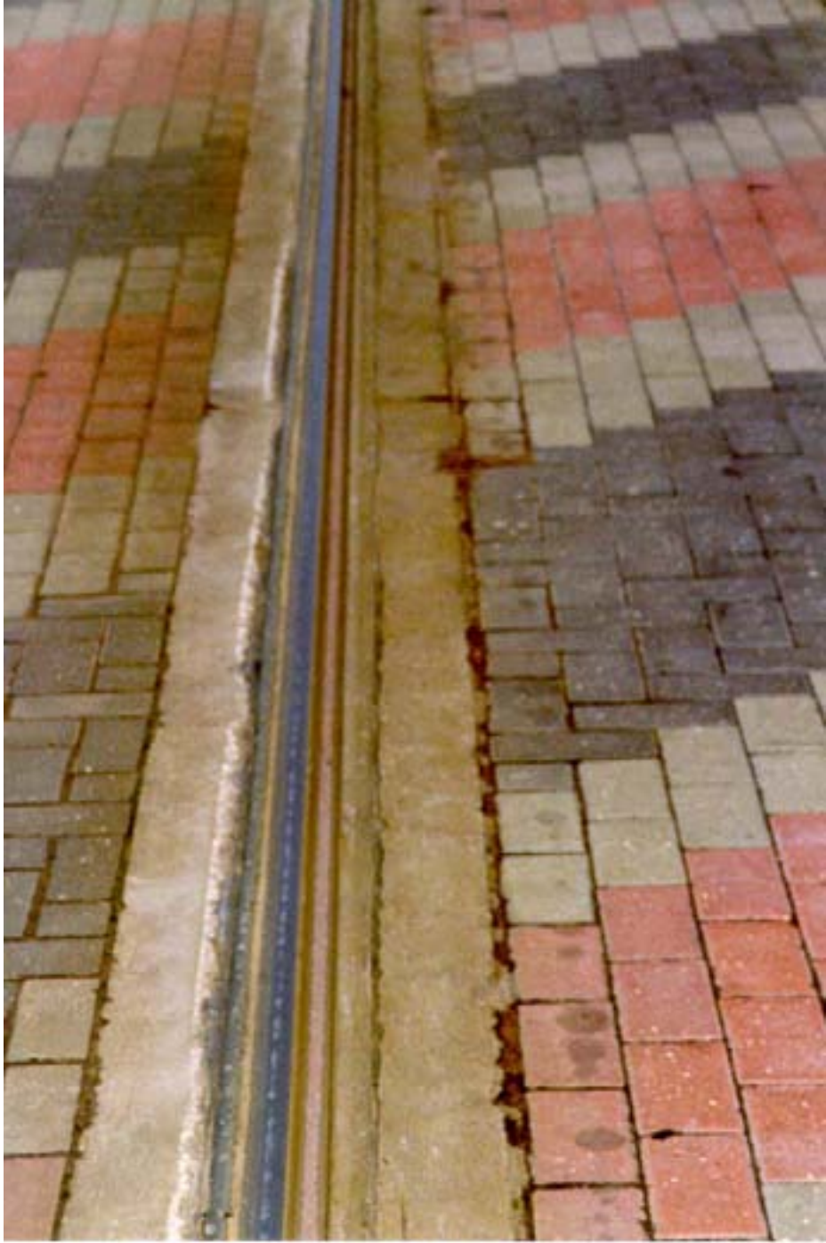
Figure 13.3 Road surface damage due to hollow wheel wear.
