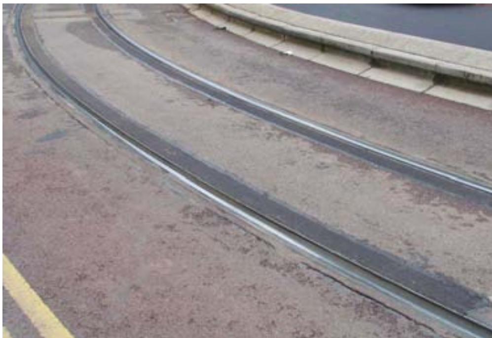
Figure 13.1 Example of curved track where rail tipping has been found
