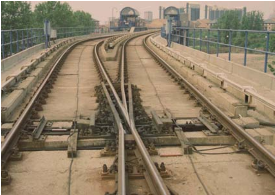
Figure 4.21 The original design of slab track swing nose turnout Docklands Light Railway
