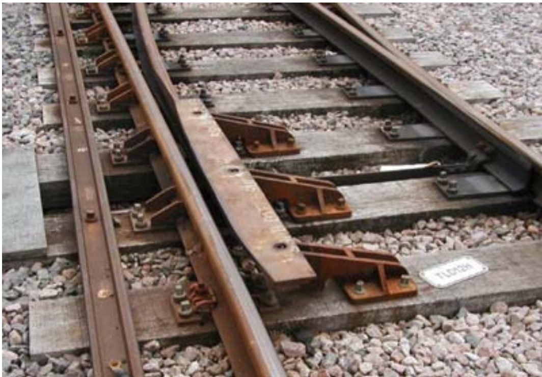
Figure 3.19 Over-rail turnout check plate at the Croydon Depot (07.08.02), Croydon Tramlink
