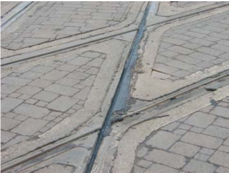
(b) Groove filled with debris
