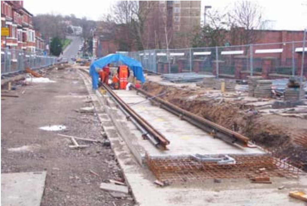
(a) Installation of rail on concrete slab (05.02.02)
