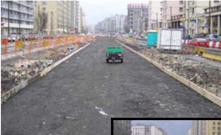
(a) Consolidated hardcore trackbed
