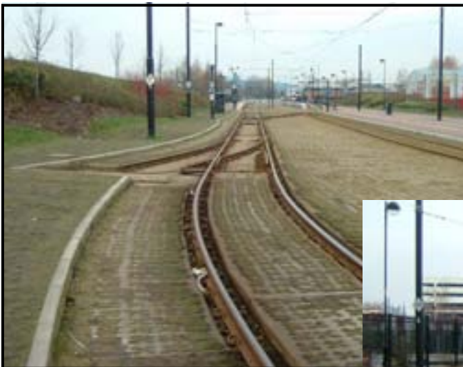
(a) Broadway Curve adjustment switch
