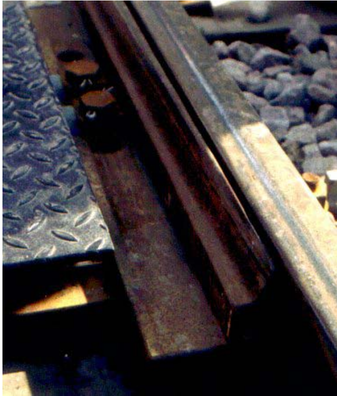
Figure 13.4 Example of a switch rail that has not been fully closed by the switch mechanism
