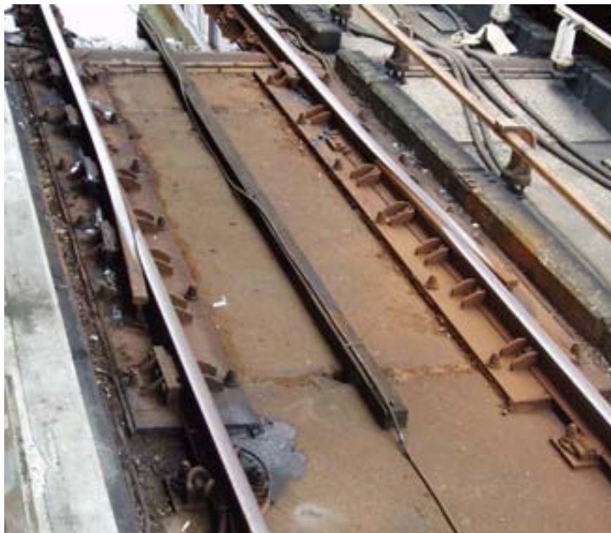
(a) 'Cologne Egg' resilient rail fastenings
