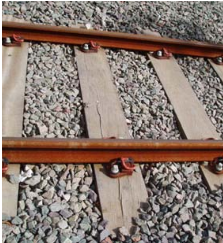
Figure 8.15 Example of track with timber sleepers in the NET Depot yard (11.09.04)
