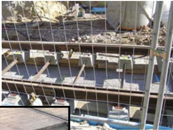
(a) Track being assembled on a concrete foundation slab
