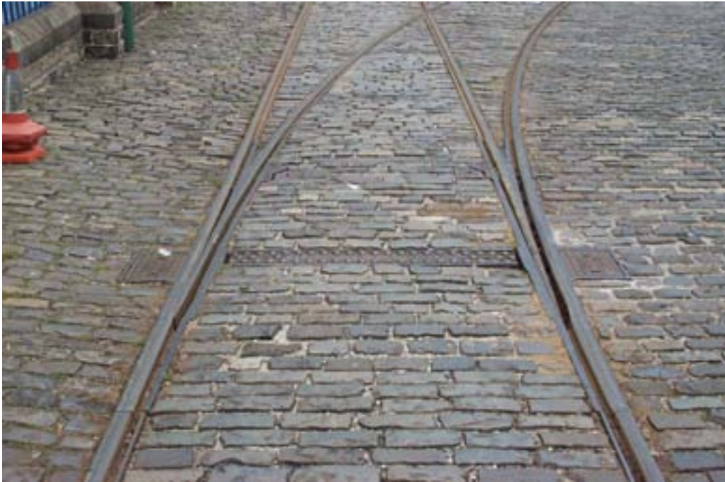
Figure 7.6 A double-bladed turnout at The National Tramway Museum
