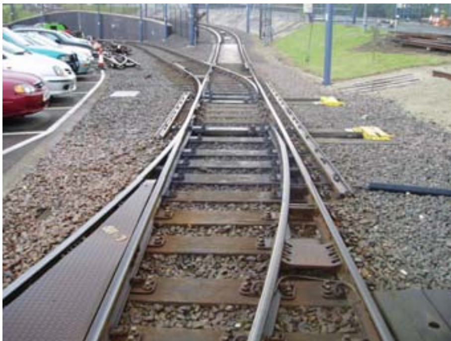
Figure 9.10 Bracing fitted to a ballasted turnout within the SYS Depot (06.10.04)
