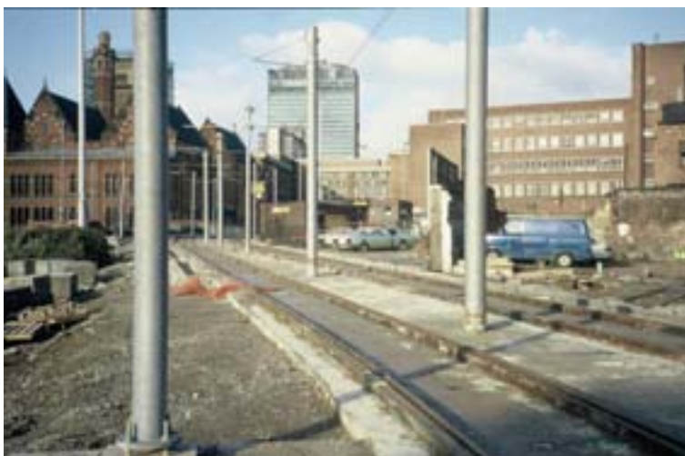
(c) Rail installed
