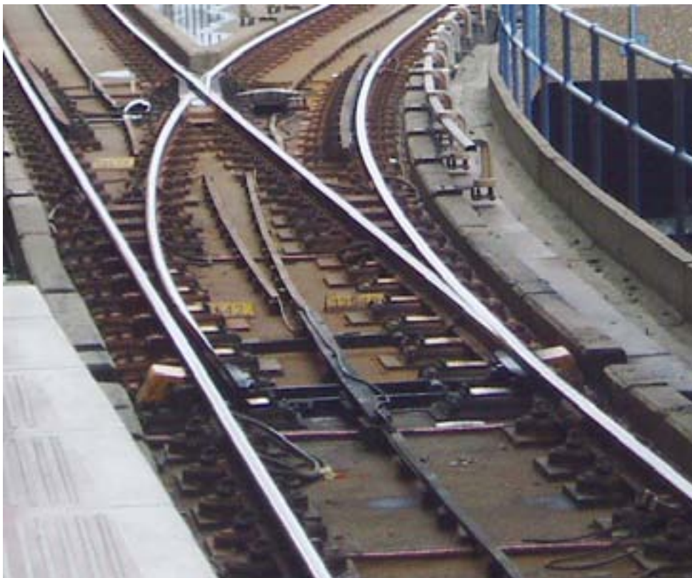
Figure 4.20 Slab track pivoted crossing nose turnout at Canary Wharf on the Docklands Light Railway (22.10.04)
