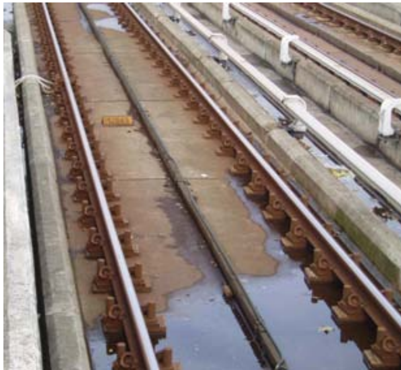
Figure 4.9 Alternative plain line slab track resilient fastenings on the Docklands Light Railway (22.10.04)
