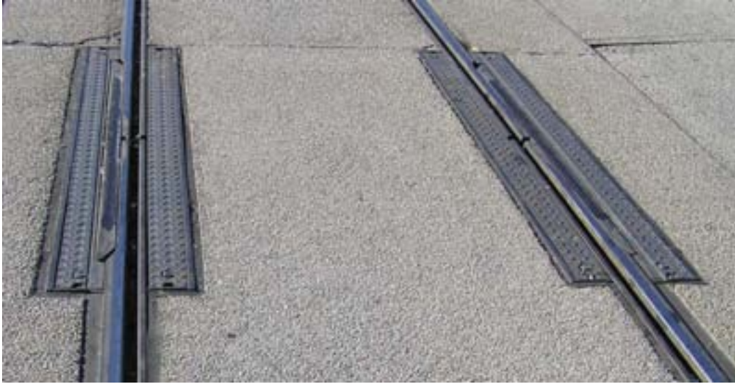
Figure 11.16 Expansion switch example, TaM Montpellier (03.03.05)
