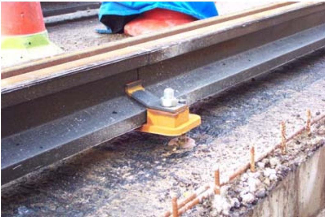
(b) Detail of fixing plate and levelling bolt (05.12.01)
