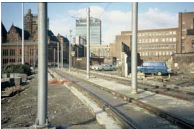
(c) Rail installed
