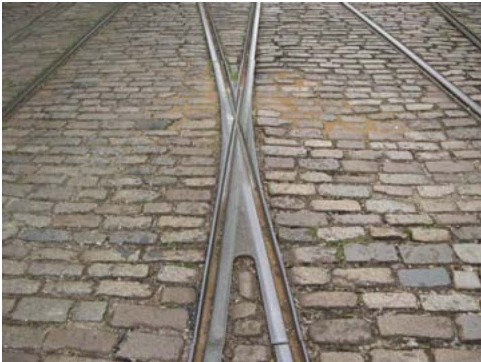
Figure 7.7 A raised groove crossing at The National Tramway Museum
