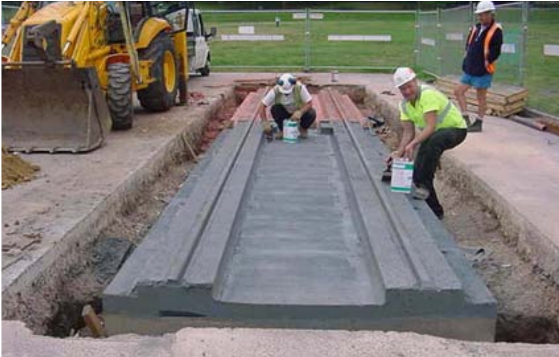
(a) Completed second stage concrete awaiting the blacktop
