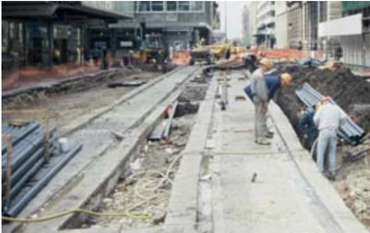
(a) Concrete track slab
