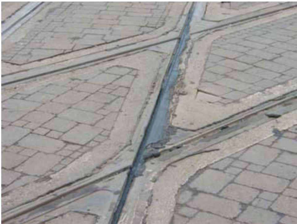
(b) Groove filled with debris
