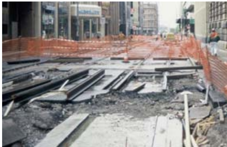
(b) Installing grooved rail
