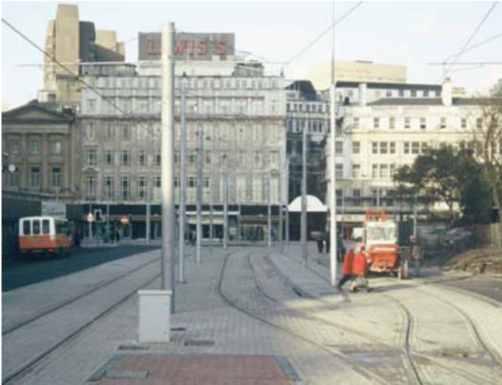
Figure 5.10 Grooved rail street track following construction, Manchester Metrolink
