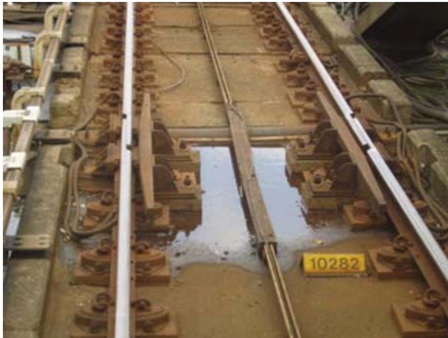
(a) 'Cologne Egg' resilient rail fastenings
