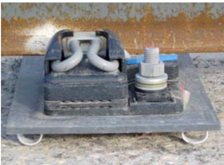
(b) Baseplate positioned for grouting
