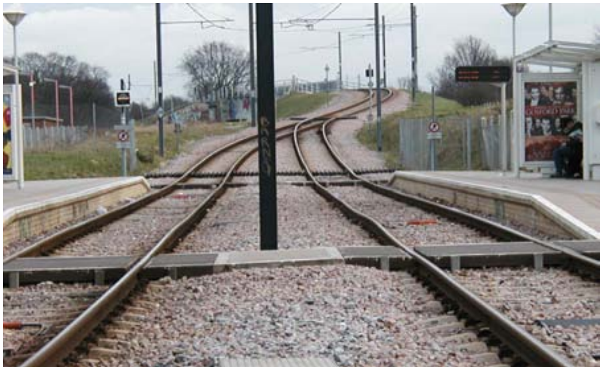
Figure 3.11 Irregular vertical track geometry at Mitcham Junction (07.08.02), Croydon Tramlink
