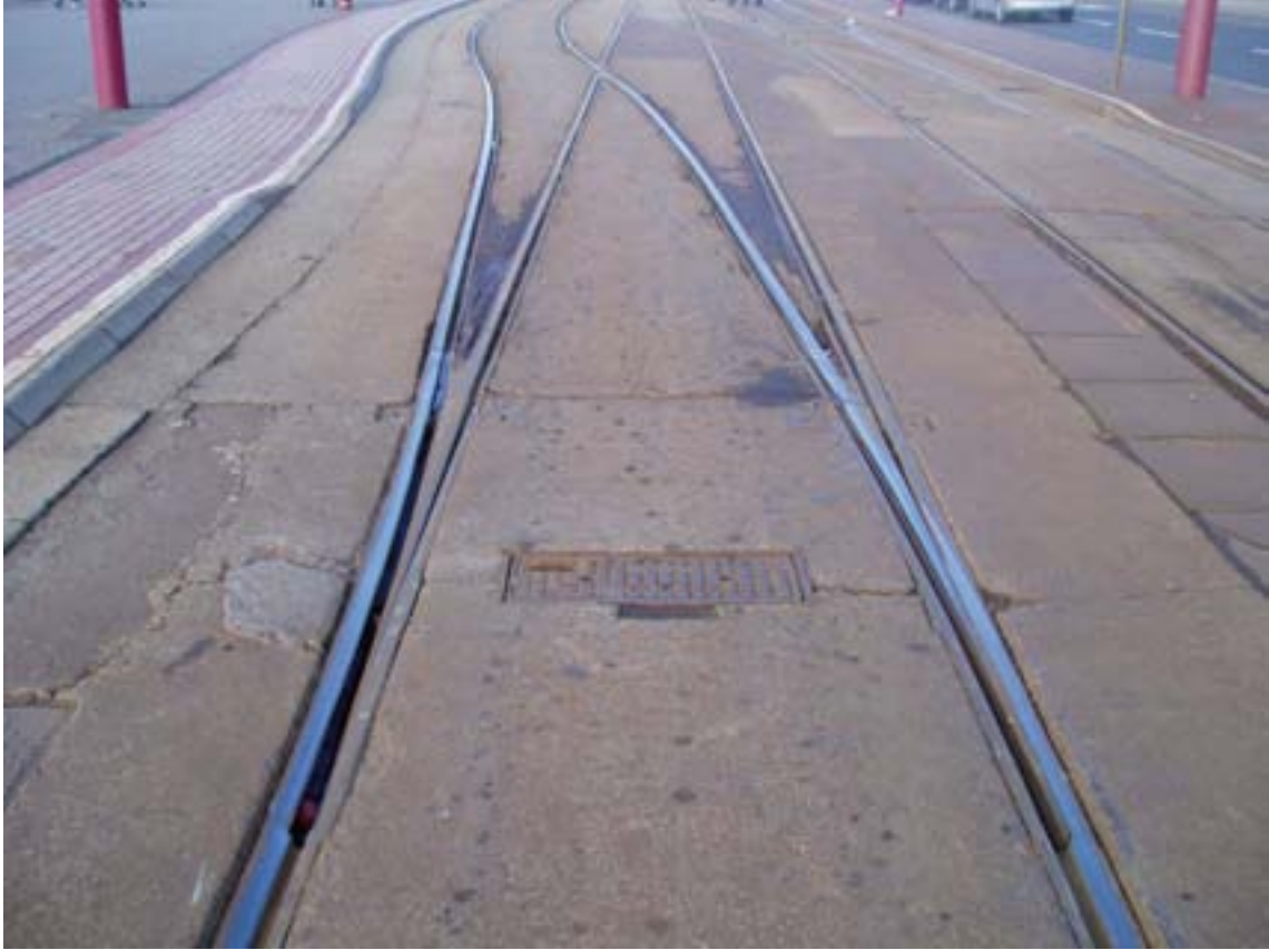
Figure 2.9 Blackpool and Fleetwood tramway grooved rail turnout (04.10.04)
