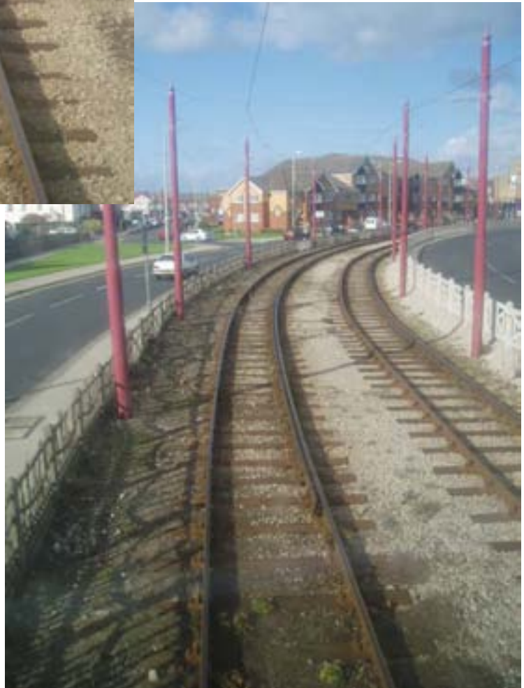
(b) Ballasted track with check rails
