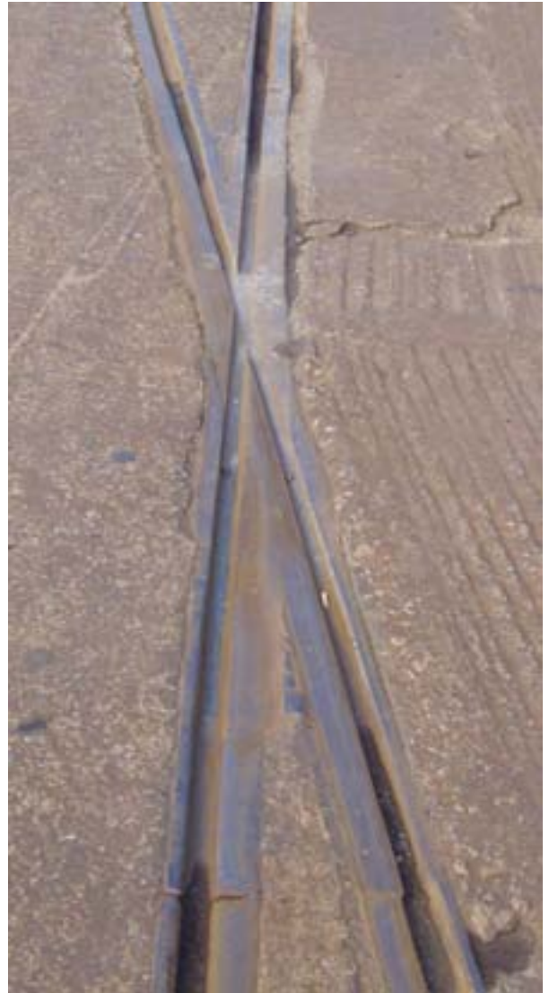
(b) Flange tip running crossing
