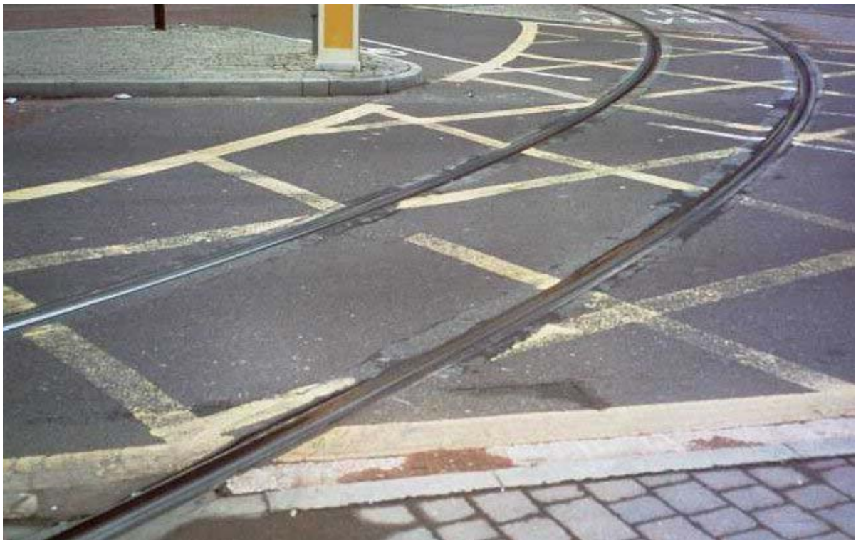
Figure 3.3 Grooved rail track at Croydon, Croydon Tramlink
