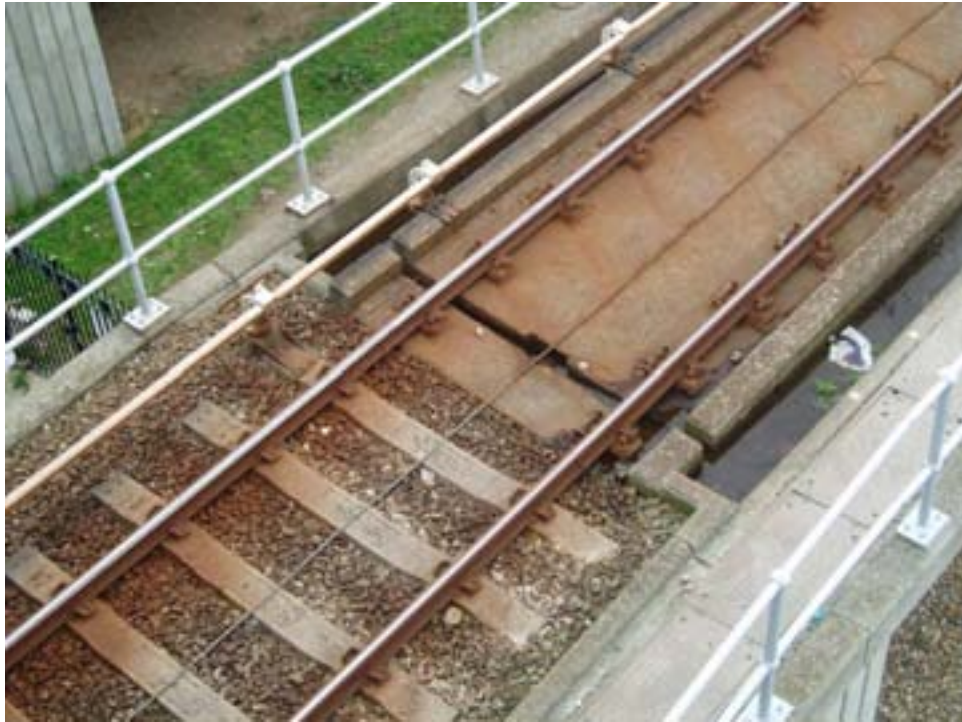
(a) A transition between ballasted and slab track on
