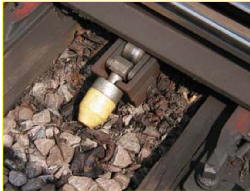
(b) Detail of a Schreck-Mieves roller support
