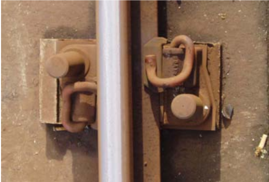
Figure 4.10 Slab track resilient rail fastening on the Docklands Light Railway (22.10.04)
