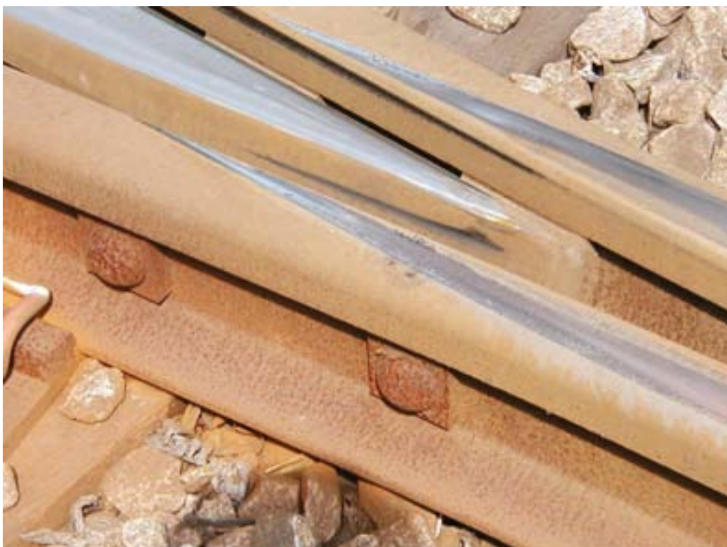
Figure 3.18 Crossing nose wear at Morden Road (07.08.02), Croydon Tramlink
