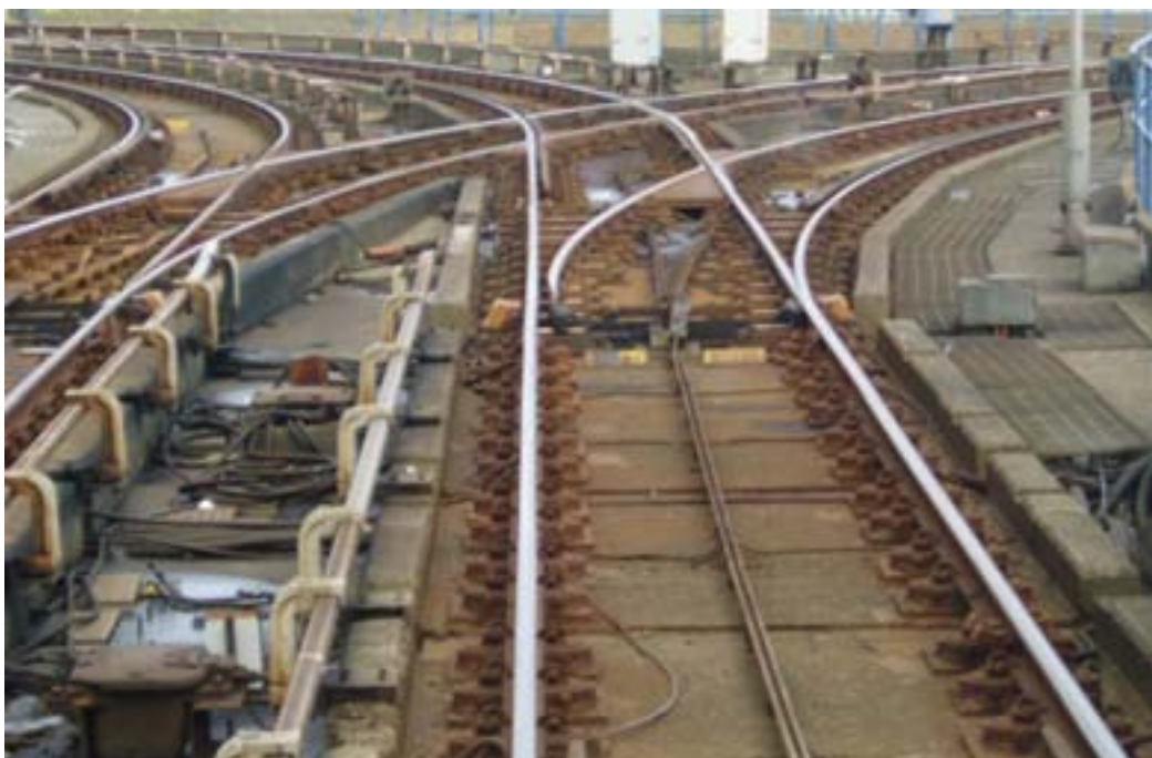
Figure 4.19 Slab track turnout at the North Quay Junction on the Docklands Light Railway (22.10.04)
