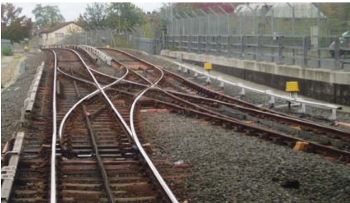
Figure 4.25 Scissors crossover at Lewisham on the Docklands Light Railway (22.10.04)
