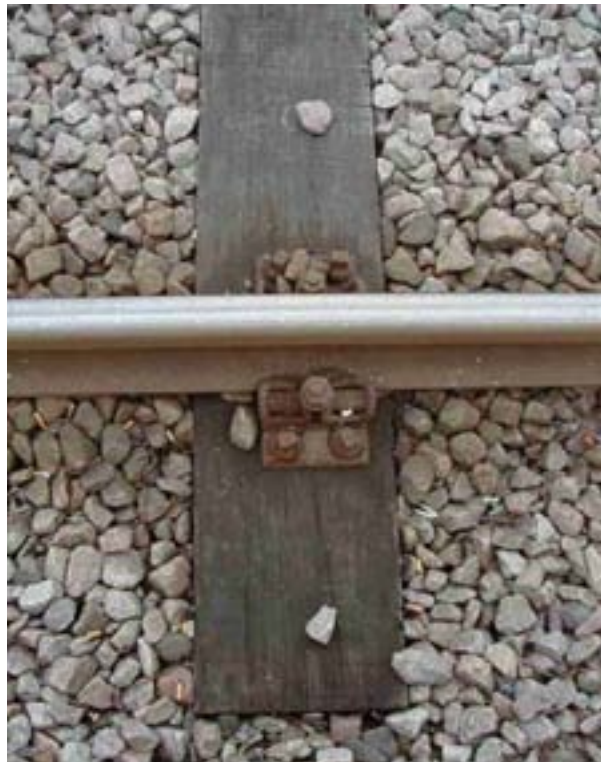
Figure 3.15 An example of ballasted track turnout construction with S 49 rail, timber sleeper and Vossloh Type KS fastenings (12.02.04), Croydon Tramlink
