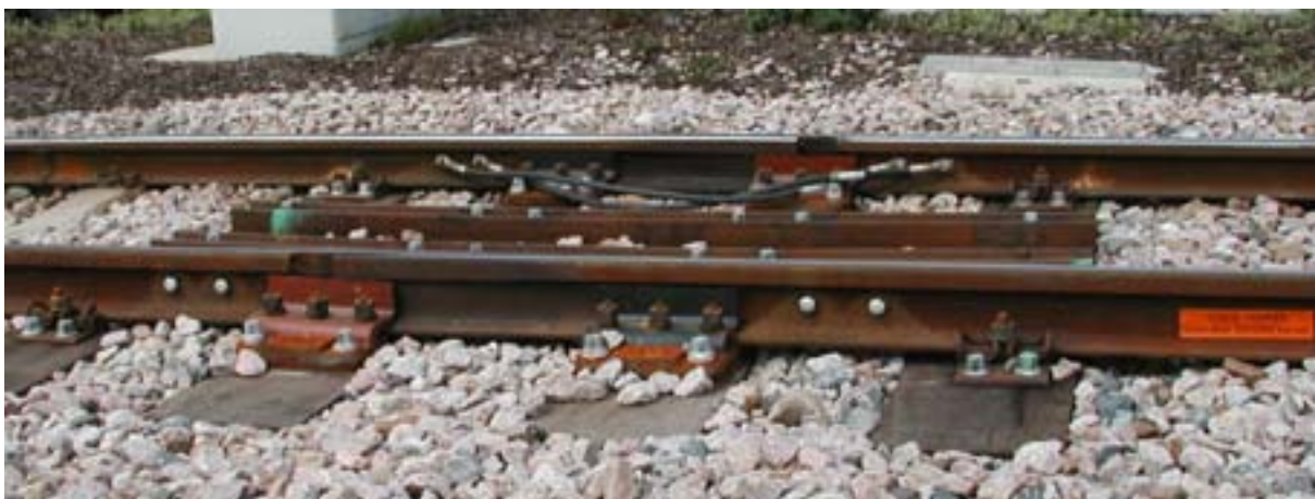
Figure 3.12 Ballasted track expansion switch (07.08.02), Croydon Tramlink
