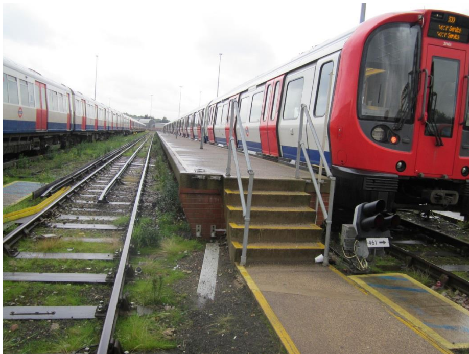
Access platform, 2.4m wide, with railed steps and conductor rails on distant side
