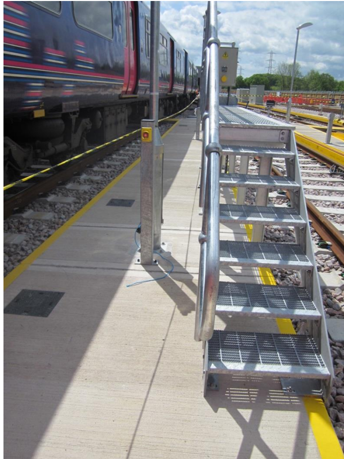
Fixed 'hop-up' platform enables safe access to cab and prevents contact with shoe-gear
