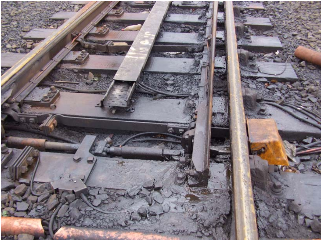
Above: Coal Spillage on Oiled Point Ends
