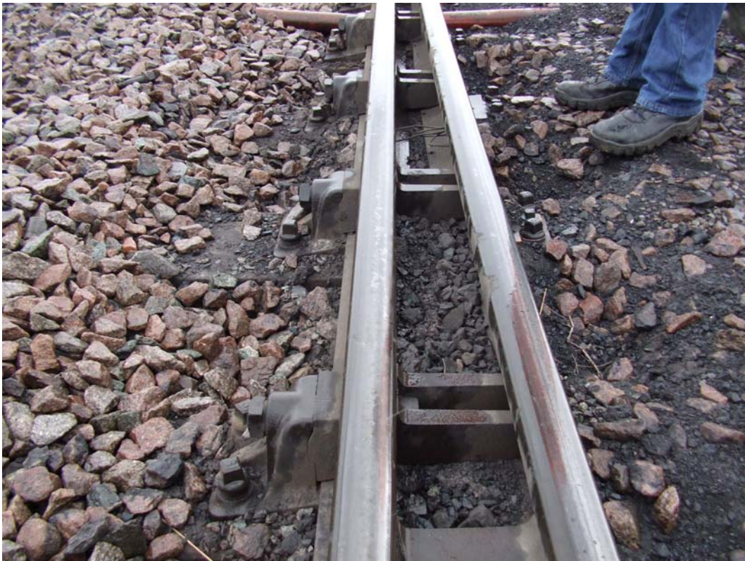
Above: Coal Spillage in moveable Switch Rail heel end Below: Severe Coal Spillage
