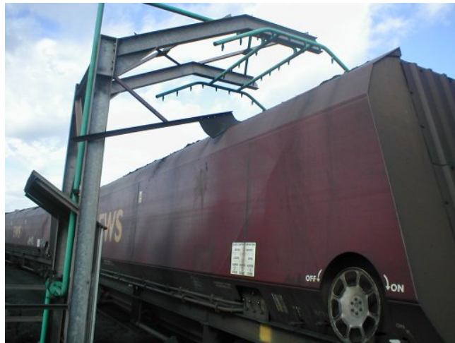
Figure 4.3.1 Spraying and Wagon Top Sweeping Gantry at Immingham
