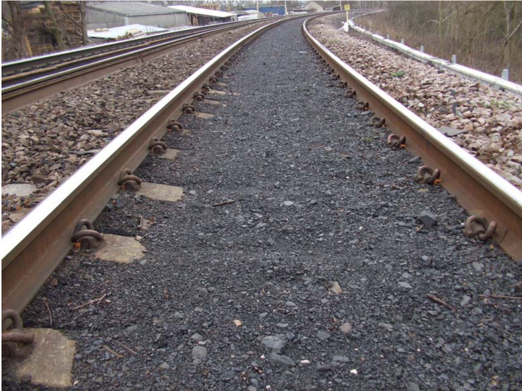
Above: Coal Spillage in moveable Switch Rail heel end Below: Severe Coal Spillage
