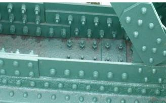
WTN/P/01/09 View of typical rivet replacement by high tensile bolts and like –for- like splice plates to restore an area where there has been a loss of section due to extensive corrosion of the bottom chord of the trusses.
