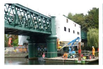
WTN/P/01/07 Encapsulated central span serviced by floating craft
