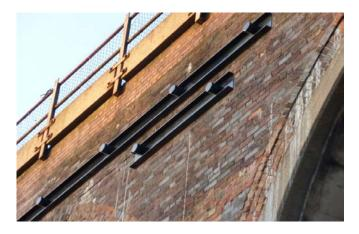
LNE/SP/02/06 Viaduct south side showing walings on span 76-77
