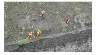
LNE/E/01/10 Record photo showing the sides of 2m wide mesh rolls being stitched together.
