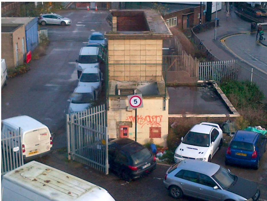
View from Over-bridge of joint ownership.
