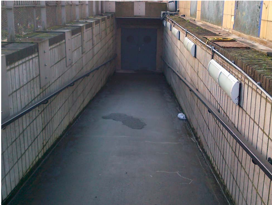
Escape ramp on developer's land
