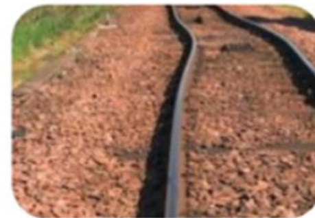
Heatwaves can cause track to buckle
