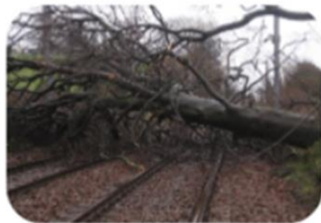
Wind can blow trees onto overhead lines and the track
