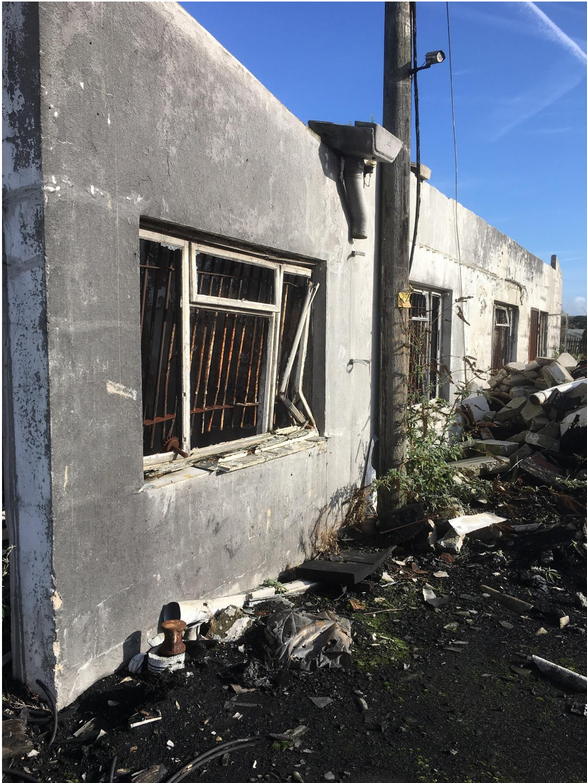
Telegraph pole? Located in the centre of the site.
