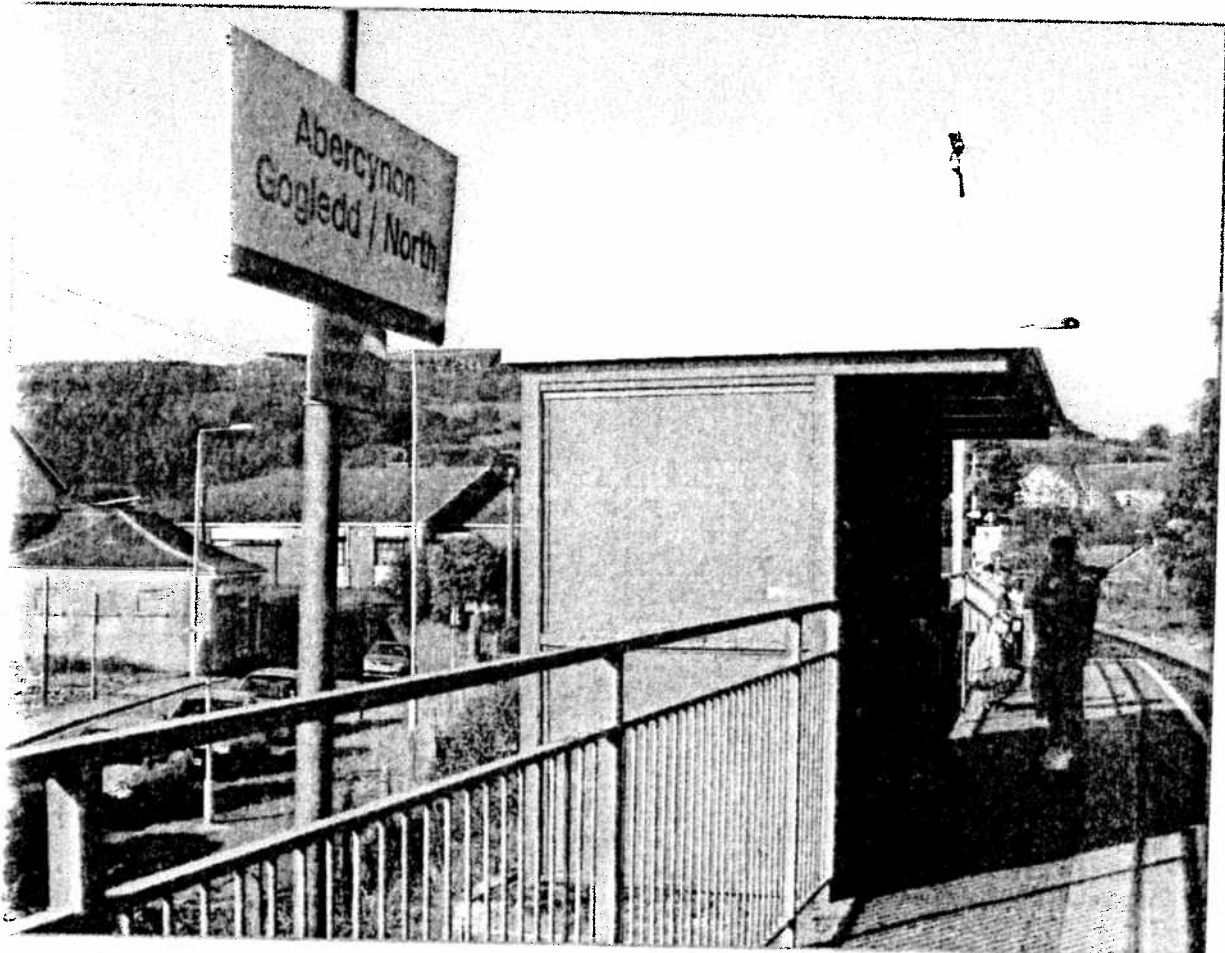
Figure 1.2 – Abercynon North Platform & Waiting Shelter
